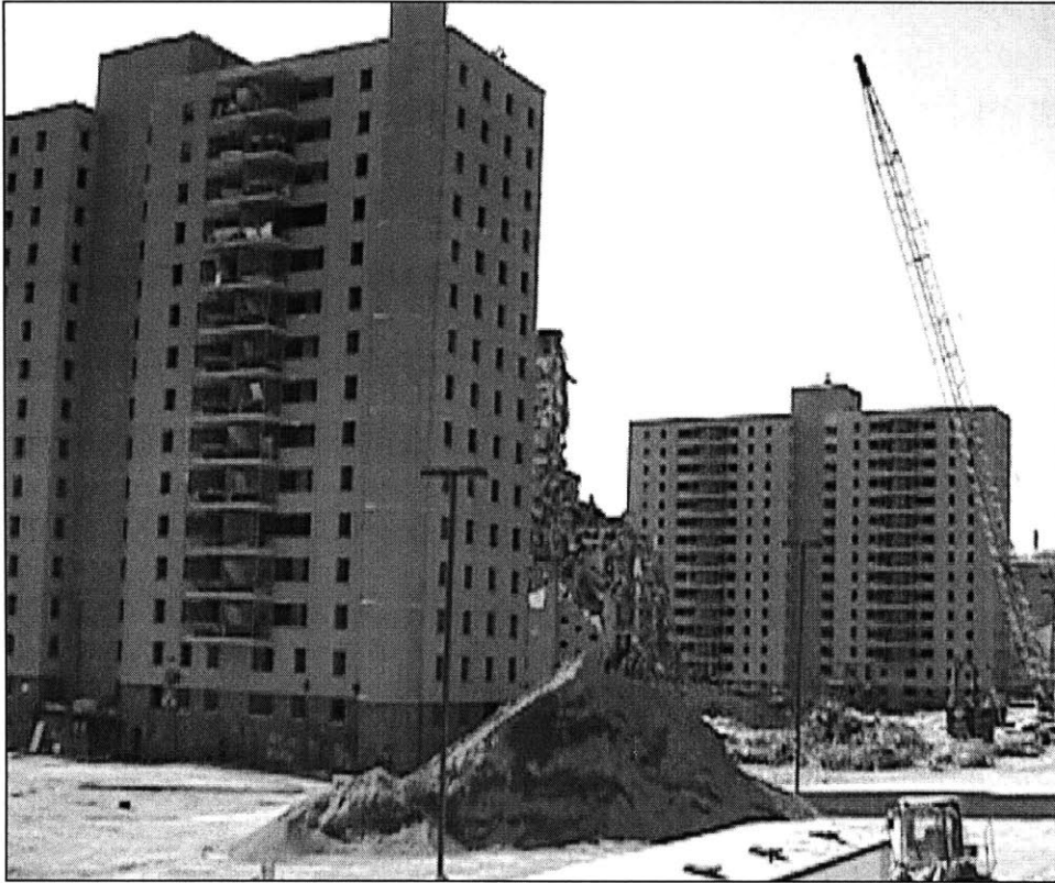
The Christopher Columbus Projects during demolition.
