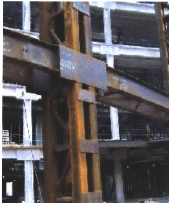
Figure 3.6 Strengthened blast connection (Source: Hardened Structures)
