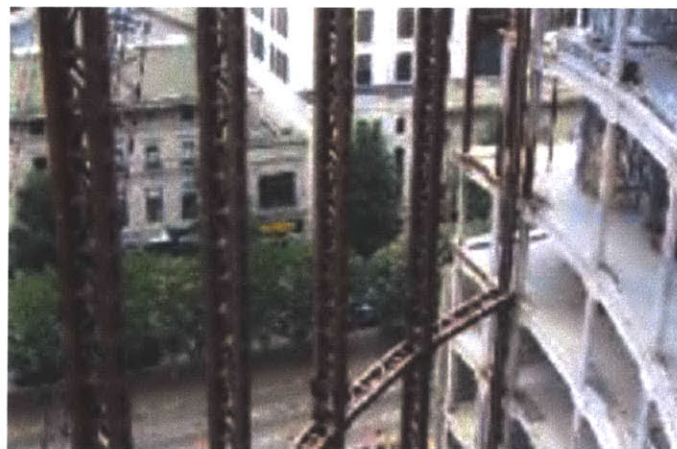
Figure 3.2 Blast curtain wall under construction (Source: Hardened Structures)
