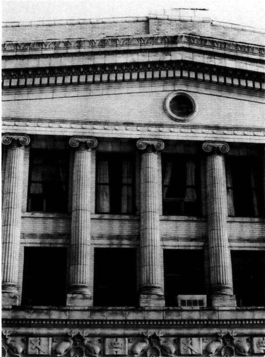
Office Windows in the Upper Facade
