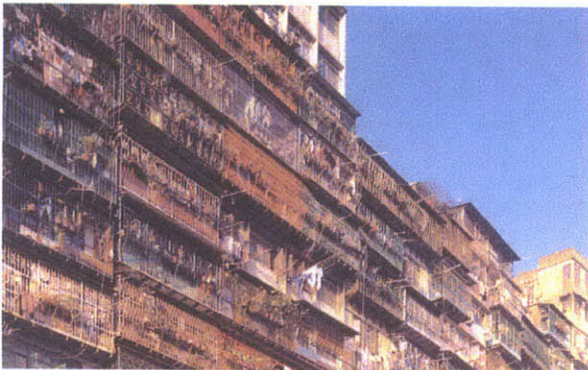
Photo of Illegal Balcony Constructions 1980's
