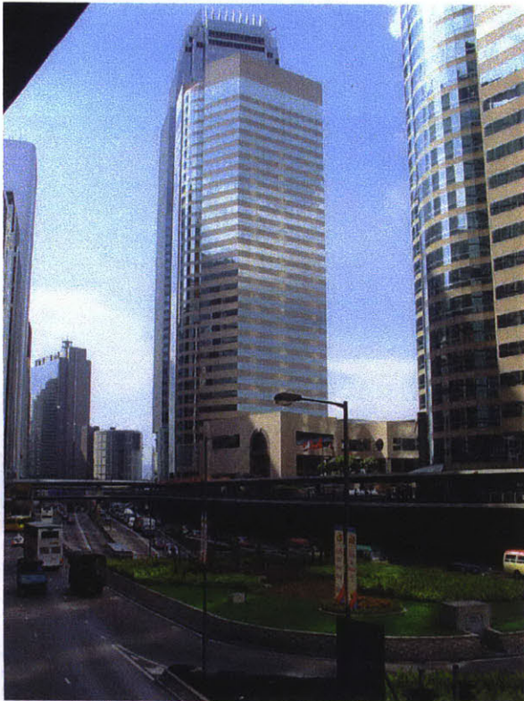
Photo of the Exchange Square Complex taken from a Section of the Elevated Pedestrian Walkway, Showing the Office Towers at the Highest Layer; Below, the Elevated Pedestrian Walkway; Then, the Roads- Connaught Road Central; and Finally, Below Ground, Hidden from View are the MTR and Vehicular Tunnels
