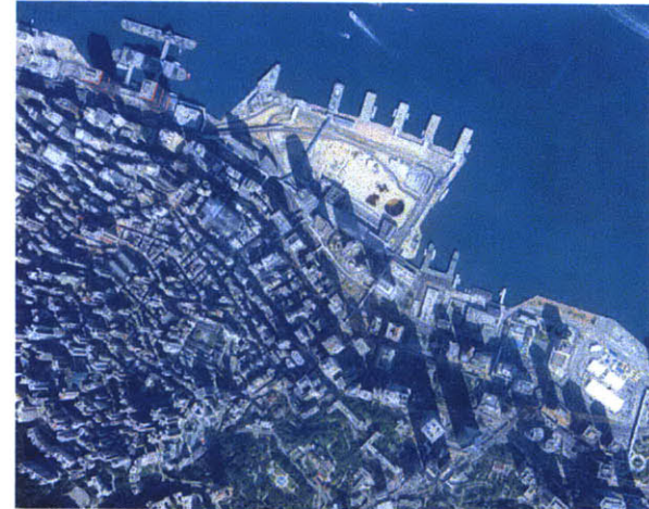
Aerial Photo of Central Showing the Reclaimed Land along the Coast Providing the Site for the new International Finance Center
