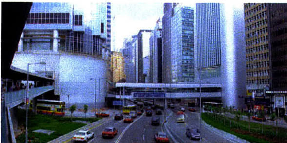
Photo of the Elevated Pedestrian Walkway Crossing Des Voeux Road Central
