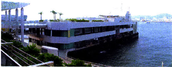
Photo of a Roof-Top Garden on One of the Ferry Piers
