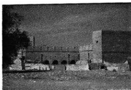
Fig.26 Concrete slab and concrete block construction. Kuwait, 1980s
