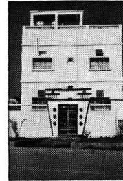
Fig.32 Entrance canopies and door details. Kuwait, 1960s
