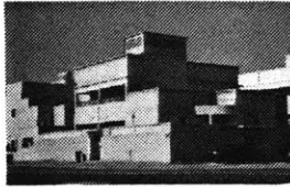
Fig.43 Terraced roofing. Kuwait, 1960s
