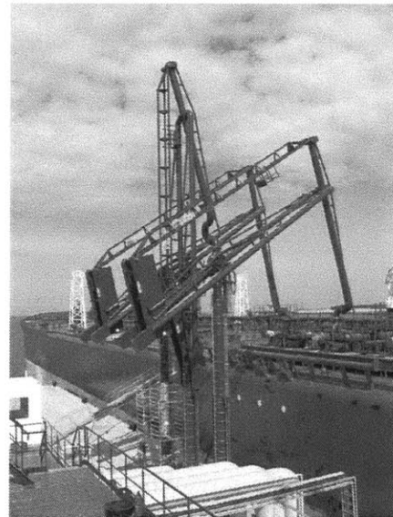
Figure 1: Loading Arms at Dock (Kanon Loading Equipment, 2011)
