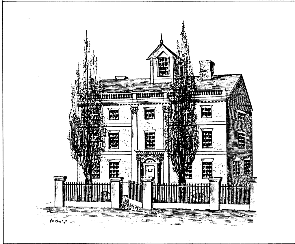
Fig 32 A Typical 18th century house. (Source: Kay, 1980.)
