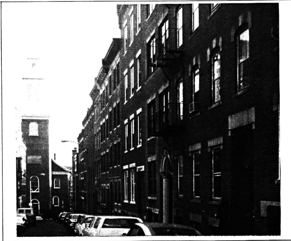
Fig 45 Series of French flats on Hull Street, most of which were built in first decades of 20th century.
