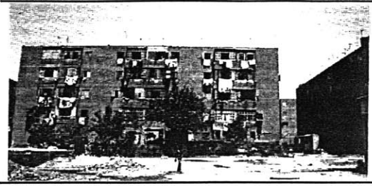
(fig. 121 ) Public Housing, Helwan, Cairo, Egypt.
