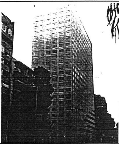
(fig. 123 ) Office building, Giza, Egypt.
