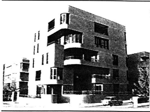
(fig. 89 ) Exterior view, residential building, Nasr city, by Bakri.
