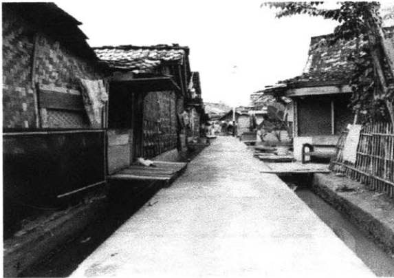
road after improvement program
