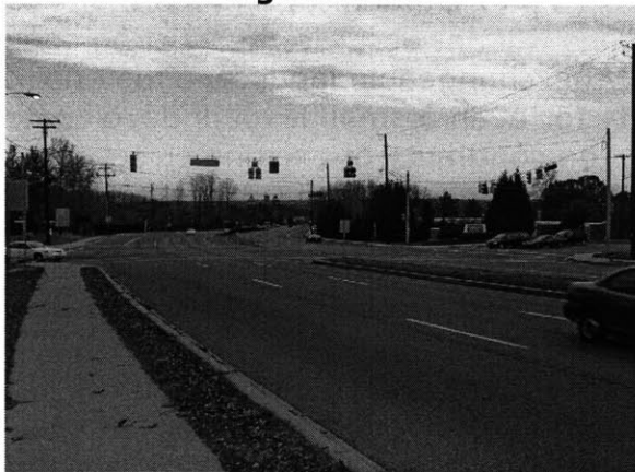
Nearby intersections and landscaping are designed for the automobile, leaving little access to the station for pedestrians.
