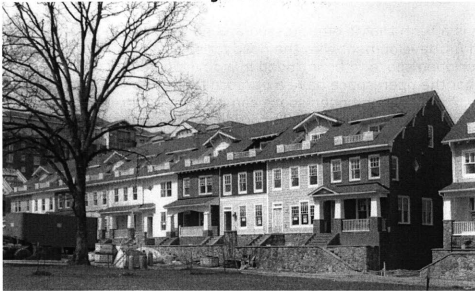
Townhouses behind the Market Common development (still under construction) face a small park.
