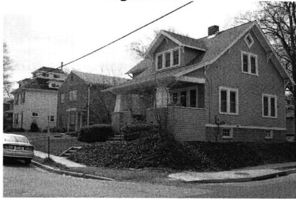
The neighborhoods near the Clarendon Station are dominated by traditional single-family residences. Most, but not all streets have sidewalks.
