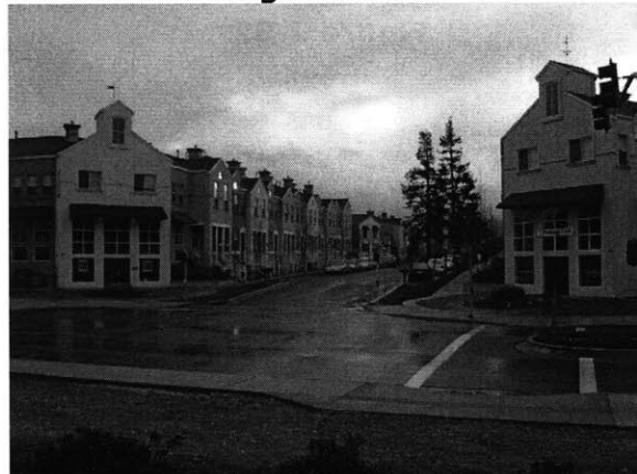
The Crossings development includes two small retail stores next to the transit station.
