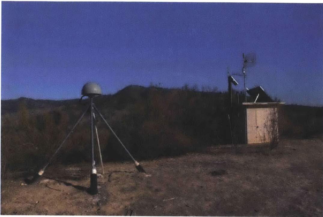
Figure 1-4. Photo of the PBO station CAND installed at Parkfield, California, in May 1999 as part of the Southern California Integrated GPS Network (SCIGN) for monitoring strain accumulation across the San Andreas Fault and deformation associated with Parkfield earthquakes. The antenna with radome (left front) is mounted on the deep drilled braced monument that consists of 5 legs (one is a vertical leg braced the others) placed into drilled holes (~10 m below the surface) and welded together. The shed houses GPS and telemetry equipment (right back). The solar panel for power supply is shown on the roof of the shed and antennas for telemetry next to the shed. Photo from http://pboweb.unavco.org/shared/scripts/stations/?checkkey=CAND
