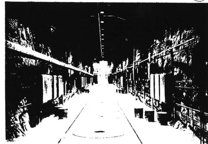
Fig. 7. A view inside a repository tunnel Department of Energy
