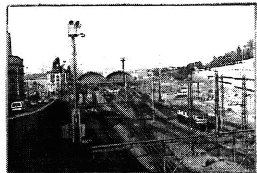
The station from the south
