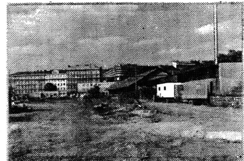
The building site, looking north-east
