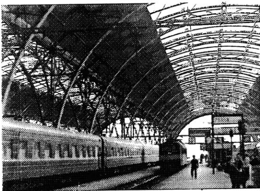
The double arch steel shed
