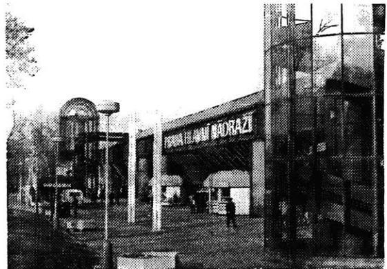
Today's main entrance to the station
