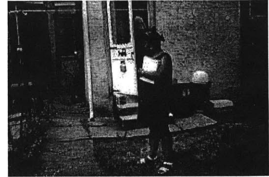
Crystal Cornitcher of the Mill Creek Coalition examines basement conditions for the "Assessing Subsidence and Flooding Conditions: Pilot Research Project," during the summer of 1999.
