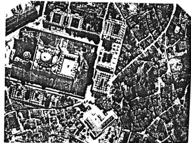
Fig.12. Aerial view of the Süleymaniye complex showing it within the fabric
