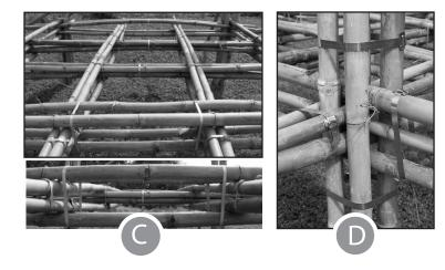
The second structure was slightly different from the first attempt. It had much stronger floor support net of primary and secondary members so that the weight is distributed more evenly. The floor members were woven together in order to provide some lateral support and the structure needed for a floor surface. The columns consisted of four main horizontal members. The structure didn't have any lateral bracing, which was the main cause for its failure.
