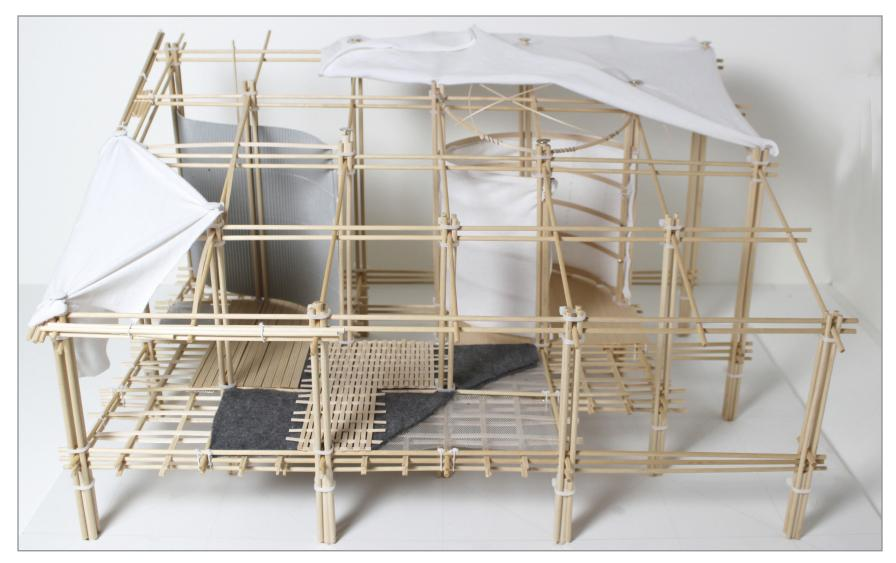
To conclude this section, the whole structure is based on redundancy. Main structural members are actually composed of several smaller poles. This redundancy in the system is necessary in order to work with the non-standard nature of the material. Several small diameter poles are easier to control than one large diameter pole. Also, the smaller members allow for the 3-d column design, which then incorporates the rest of the structure and enclosure of the house.
