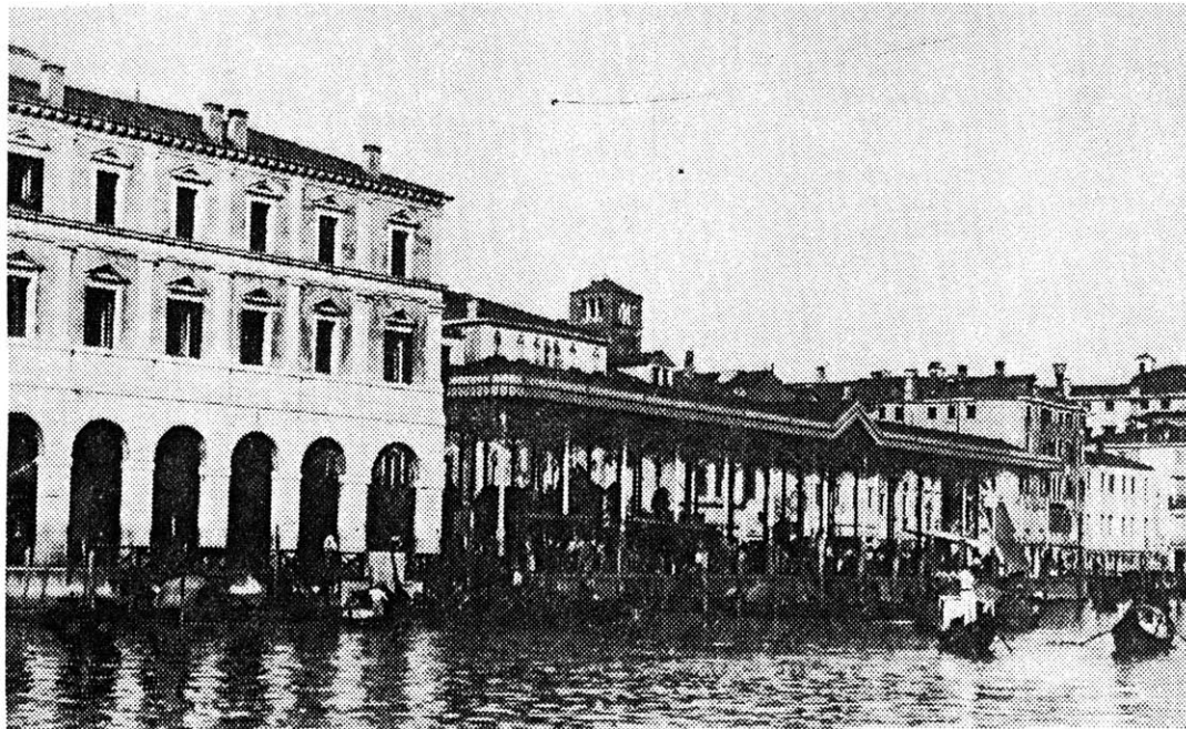
2. Market area showing Forcellini's metal-roofed market, 1884
