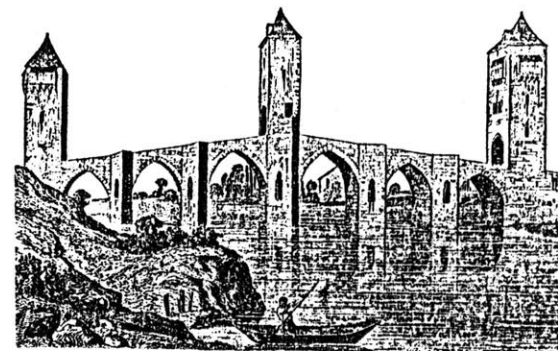
Bridge of Valentre Cahors, France Fig. 23
