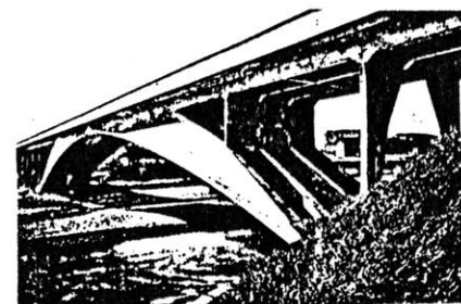
Thur Bridge Fig. 72
