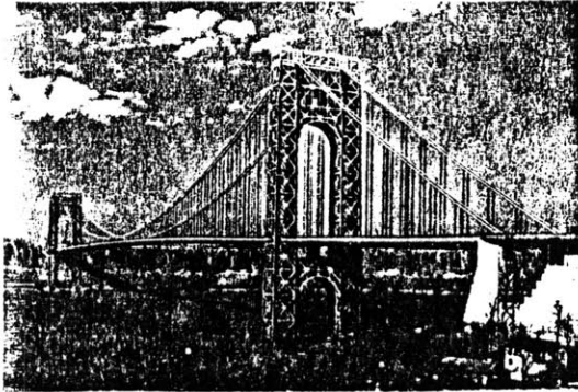
George Washington Bridge Fig. 16
