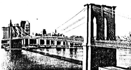
Brooklyn Bridge Fig. 17
