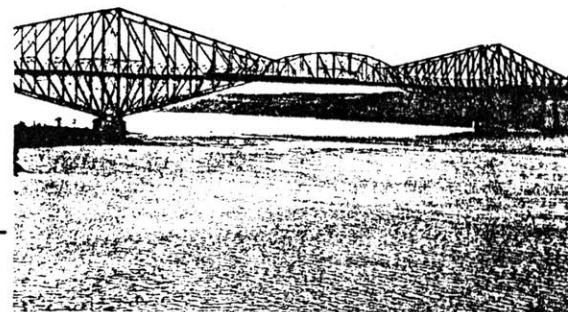
Quebec Cantilever Bridge Quebec 1917 Ralph Modjeski Fig. 14
