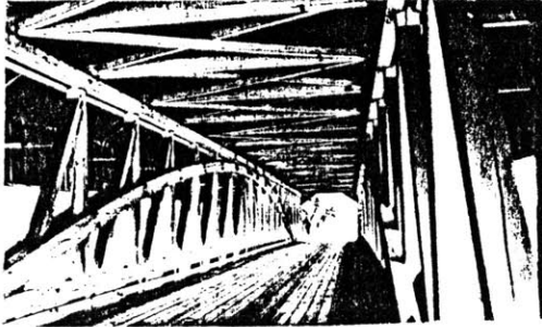
"Burr-arch" truss Fig. 35
