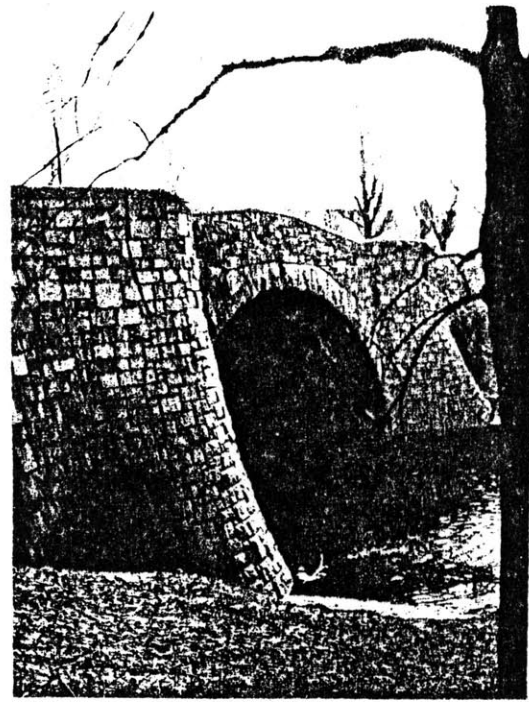
Fenway Bridge, Boston Massive stone bridge H.H. Richardson Fig. 18
