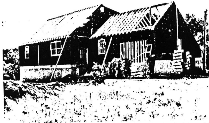
A precut house comes with bundles of essential parts and lumber sized for quick nailing in place. New England Components/Techbuilt.
