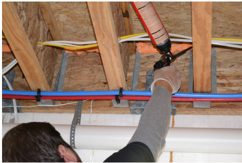
Figure 4.10. Sealing the rim joists and the plumbing penetrations in the loose house did not greatly affect the flow rates during the blower door test.
