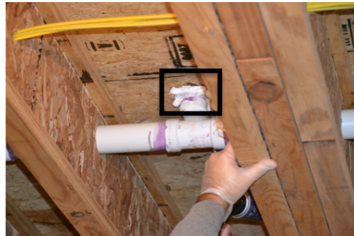
Figure 4.10. Sealing the rim joists and the plumbing penetrations in the loose house did not greatly affect the flow rates during the blower door test.
