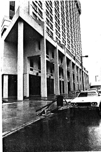
Logan Circle East (324-unit life-care facility)
