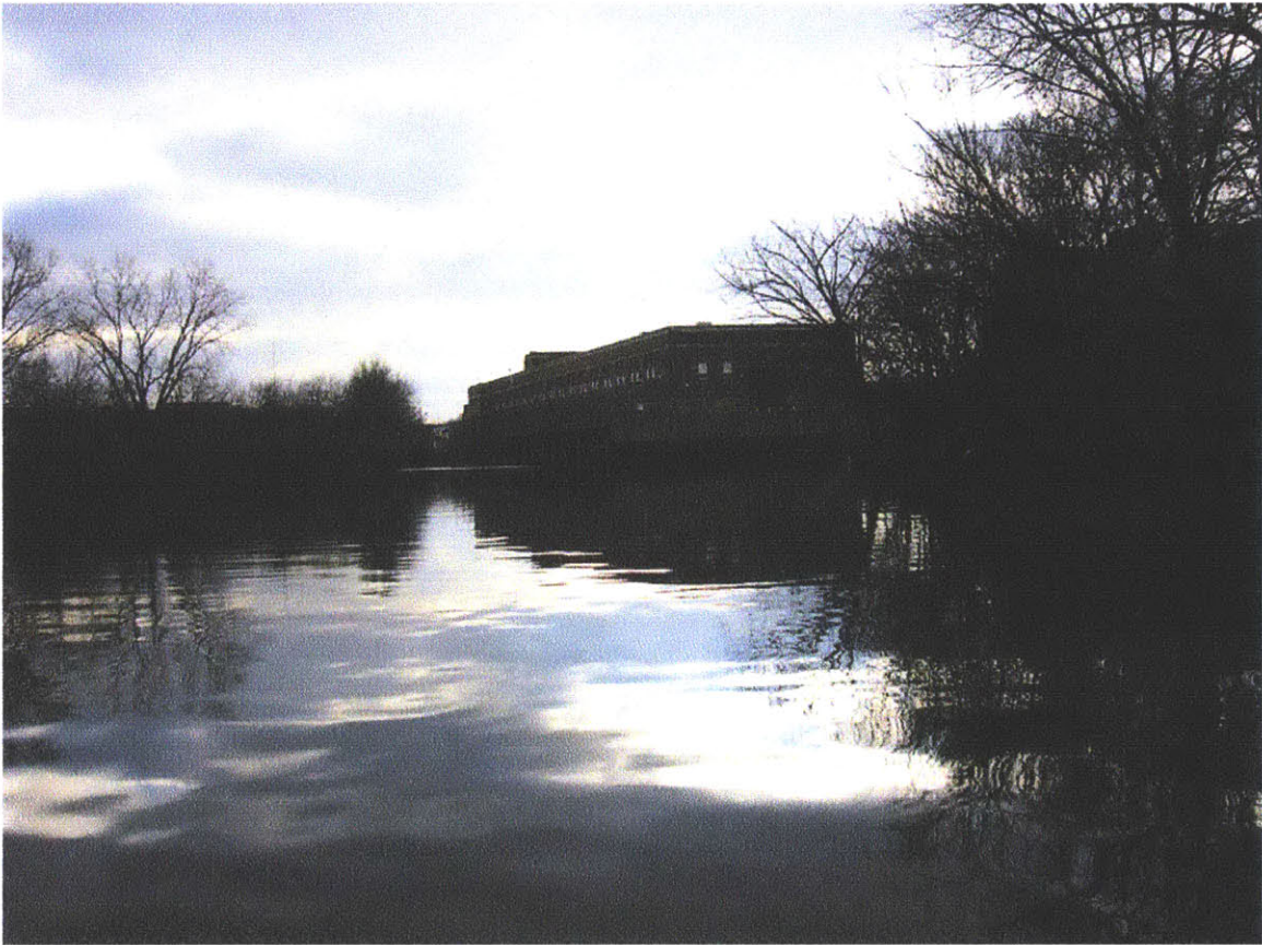
Figure: Existing Racine Avenue Pumping Station
