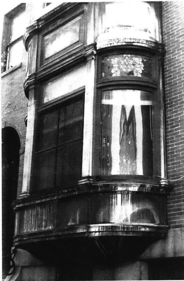
The patina of a copper-clad bay window (EVD)
