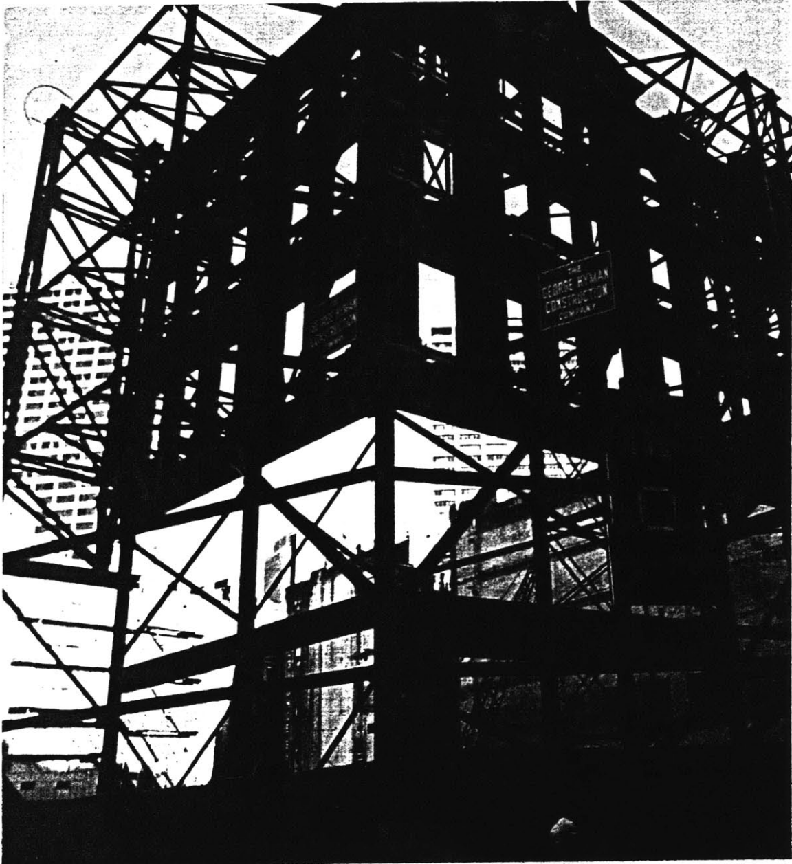
The Kennedy Store renovation: Preservation of the upper three stories of the 1873 facade.
