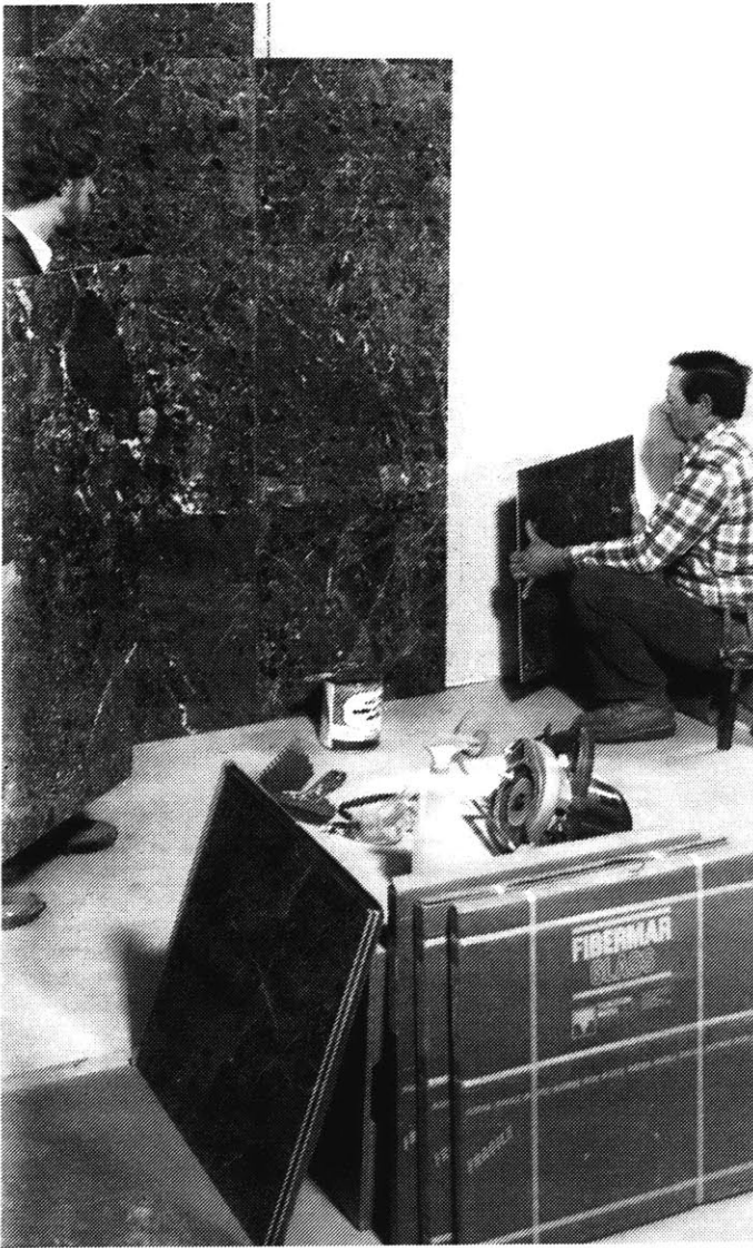
Carpenters installing marble tile with adhesive
