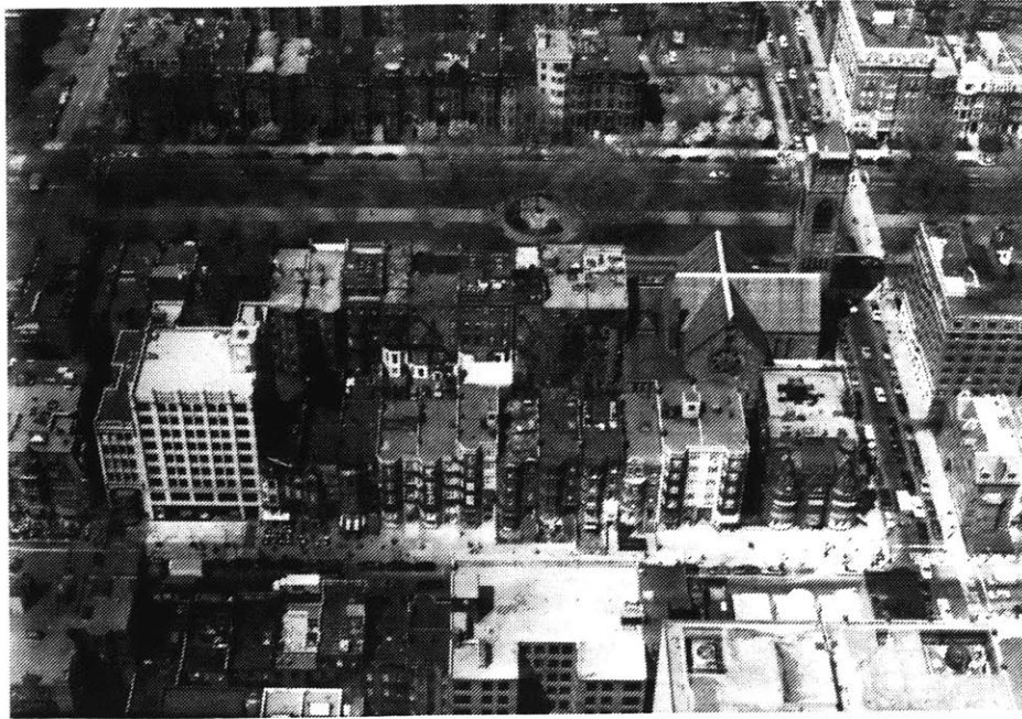
Aerial Photograph of Newbury Street, Boston - Notice the thinning nature of the facades which fashion the surface image of the individual structures. Image is only skin-deep. (EVD)
