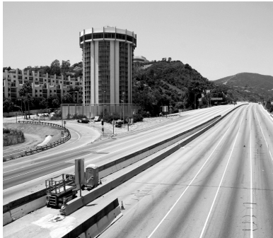
Carmageddon, 2011 Photo of I-405 Freeway and Hotel Angeleno in Brentwood, Los Angeles, during the 2011 closure of the Sepulveda Pass. mehdibouquaphotos.blogspot.com
