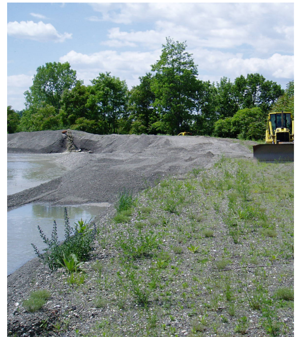
Image 5 :: An example of an Upland Disposal Site, (Canal Corp, 2012)
