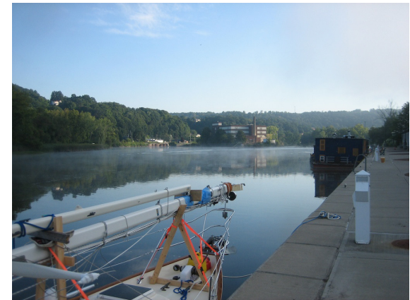
Image 4 :: An example of a Terminal Wall is shown on the right side of the photograph, (Talisman, 2011)
