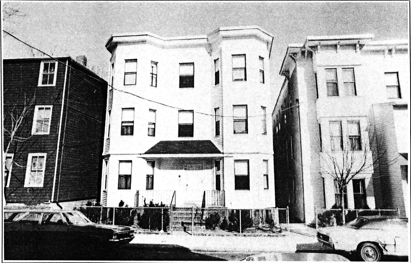
FIGURE 25: Cambridge Turnkey-III Low-Income Home Ownership Program, 47 Lopez Street. Six low-income families reside here as a result of this C.H.A. program.
