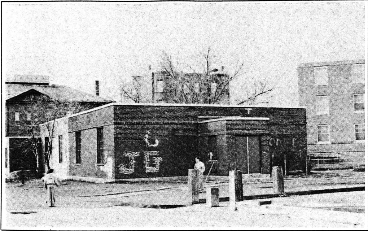
FIGURE 10: New Towne Court, Gymnasium. Closed for nearly ten years, the building shows signs of abuse and neglect.
