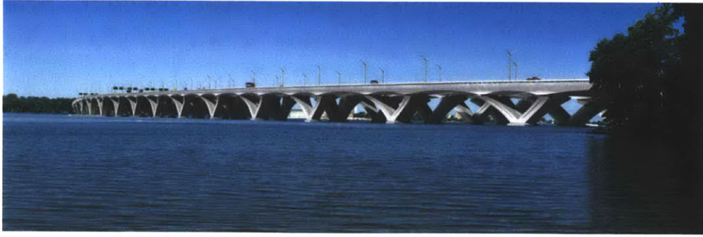
Figure 4.9 Woodrow Wilson Bridge Design Competition, Winning Design by Parsons Transportation Group (Entry B); Source: (Selection Panel Renderings Booklet 1998)
