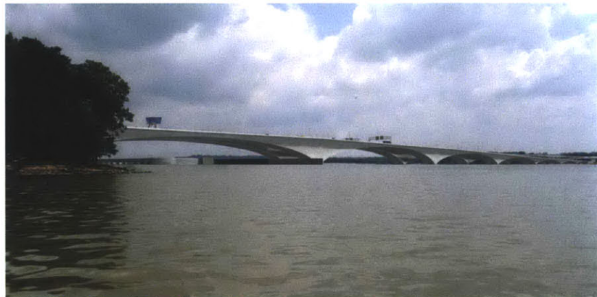
Figure 4.7 Woodrow Wilson Bridge Design Competition, Entry T - HNTB Corporation; Source: (Selection Panel Renderings Booklet 1998)
