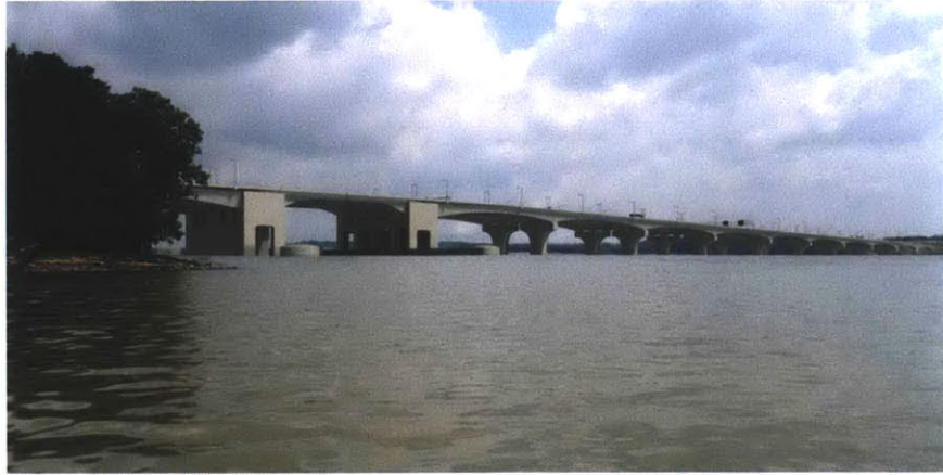
Figure 4.6 Woodrow Wilson Bridge Design Competition, Entry Q - Figg Engineering Group/Johnson, Mirmiran & Thompson; Source: (Selection Panel Renderings Booklet 1998)
