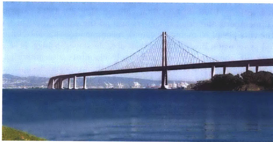
Figure 3.24 San Francisco-Oakland Bay Bridge, MTC Recommended Single Tower SAS design; Source: SAS photo simulation from Caltrans/MTC
