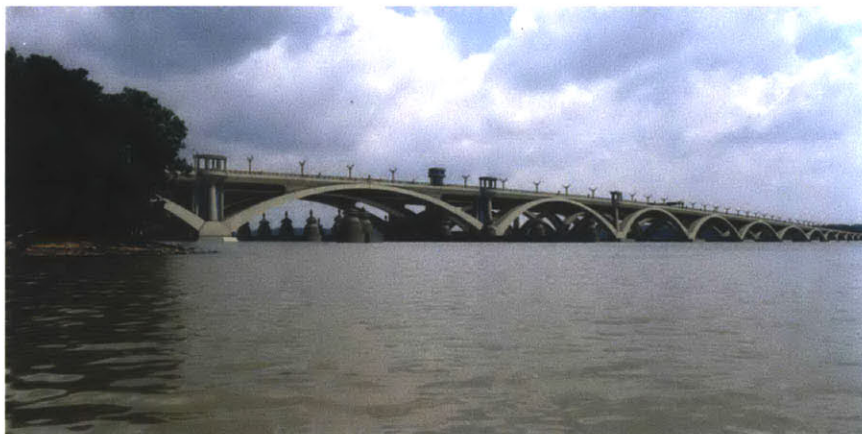
Figure 4.5 Woodrow Wilson Bridge Design Competition, Entry D - T.Y. Lin International ; Source: (Selection Panel Renderings Booklet 1998)
