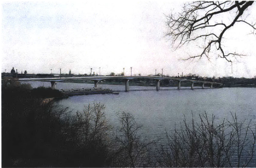
Figure 2.6 Severn River Bridge Design Competition, Entry F - Arvid Grant and Associates; Source: (Kurdle 1990)
