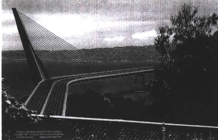
Figure 3.15 "Astaneh-Black" Steel Single Tower Curved Bridge by Professors Abolhassan Astenah-Asl and R. Gary Black of U.C. Berkeley; Source: (Frick 2005)
