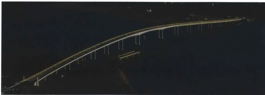
Figure 2.7 U.S. Naval Academy Bridge design competition winning entry by Grenier, Inc ; Source: (Mastaglio 1996)
