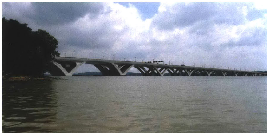
(Figure 4.3 Woodrow Wilson Bridge Design Competition, Entry B - Parsons Transportation Group; Source: (Selection Panel Renderings Booklet 1998)
