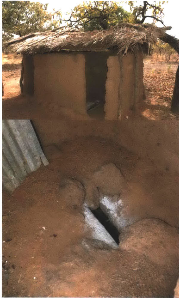
Figure 33: A local latrine built by the members of Juo-Sogon (above) and the inside slab made of mud and logs (below)
