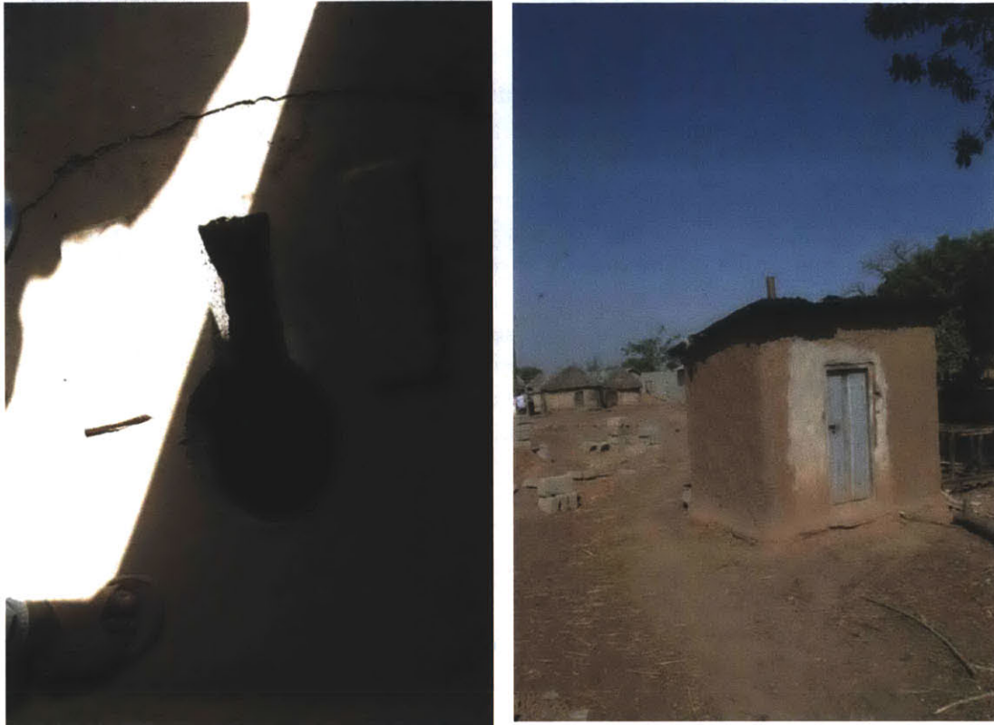
Figure 25: One of the Zagyuri latrines (right) and one of the concrete slabs provided by the NGO (left)
