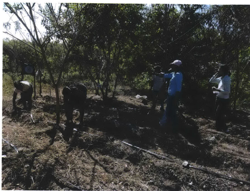
Figure 5.7: Laying the drip lateral. Photo: Susan Kinne (2012)
