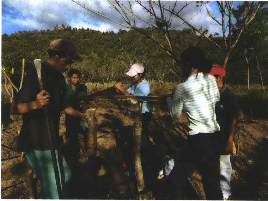
Figure 5.9: Creating a table to elevate the 33 gallon bucket. Photo: Susan Kinne (2012)
