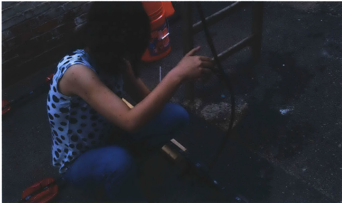
Figure 6.4: Pumping the system to start the flow of water from the water bag to the drip laterals. Photo: Lisa Johnson (2012)
