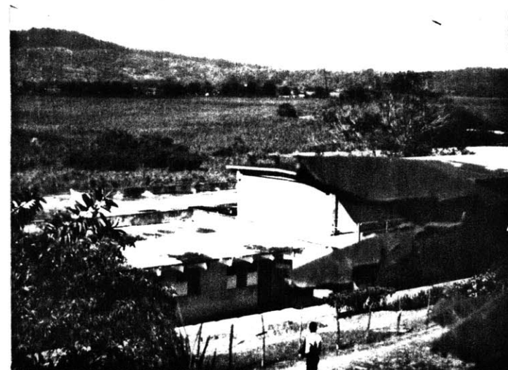
View of R.C.D.C. Site adjacent to school
