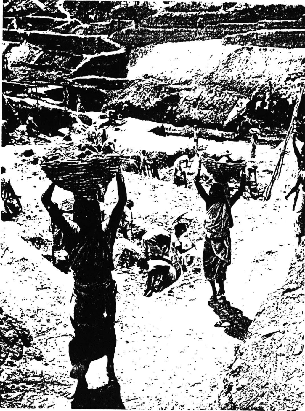
Figure A.1 Use of head baskets to carry excavated material (India)
