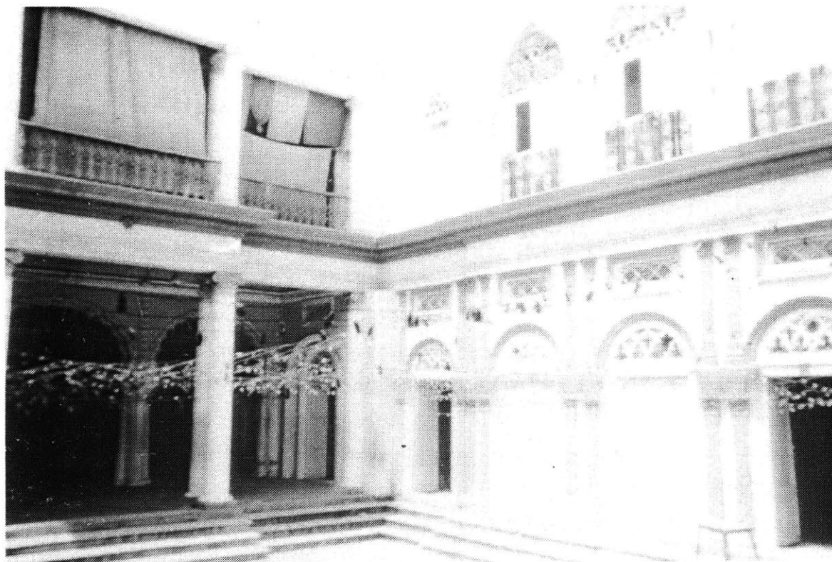
The central courtyard.
