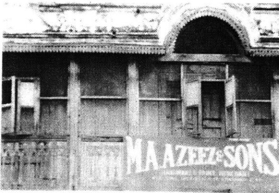
Facade treatment in old buildings.
