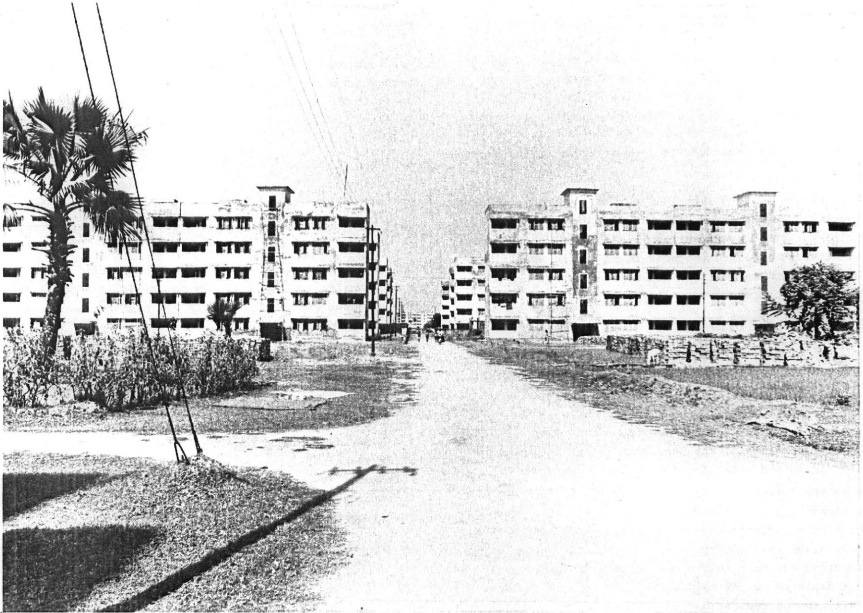
Public housing for low income groups in Dhaka. Note the abundance of left over spaces and wide streets without specific utilization, which is a waste of land and multiplies problems of control, maintenance and operation of public spaces. Photo : A.S.M. Ismail
