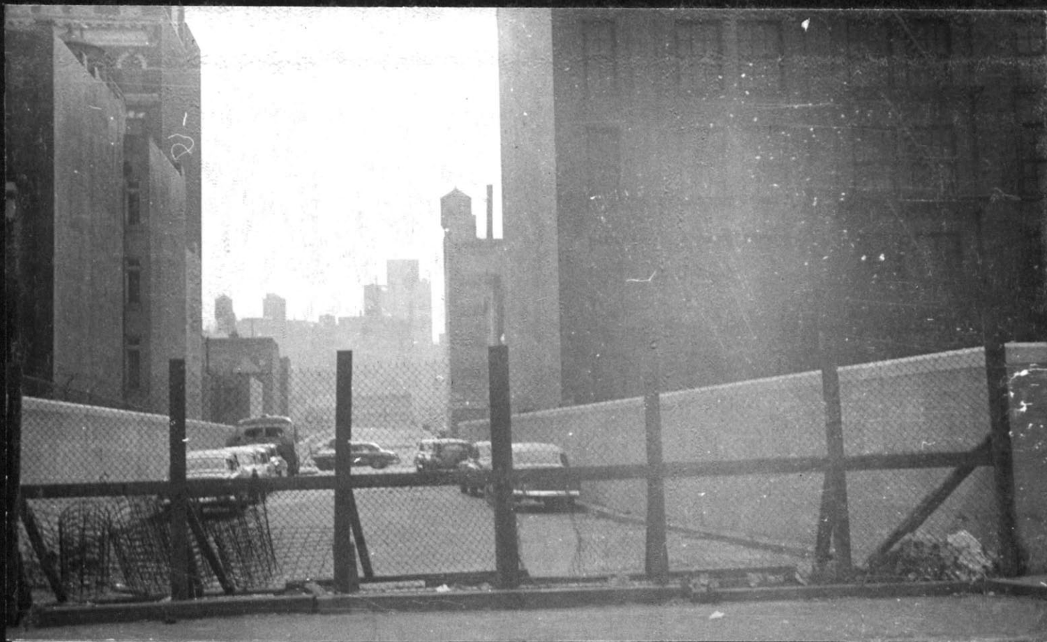
LOOKING SOUTH ALONG NEW APPROACH TO QUEENSBORO BRIDGE
