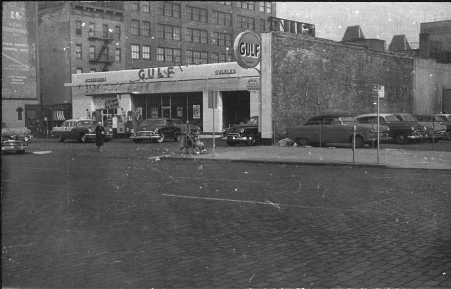
THE SITE AS SEEN FROM WEST SIDE OF SECOND AVENUE
