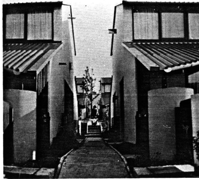
Above: Edward Cullinen's sensitive use of modern building materials adds life to this housing complex.
