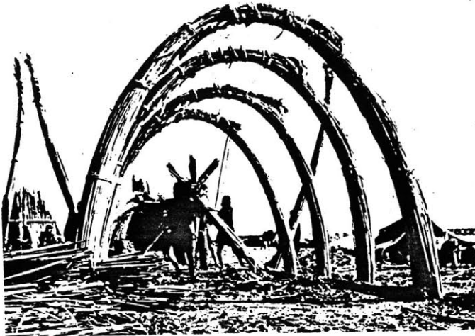
Left: Construction method in Southern Iraq. The form results from spatial use needs, the technical means available, and the natural characteristics of the river reed used as the building material.
