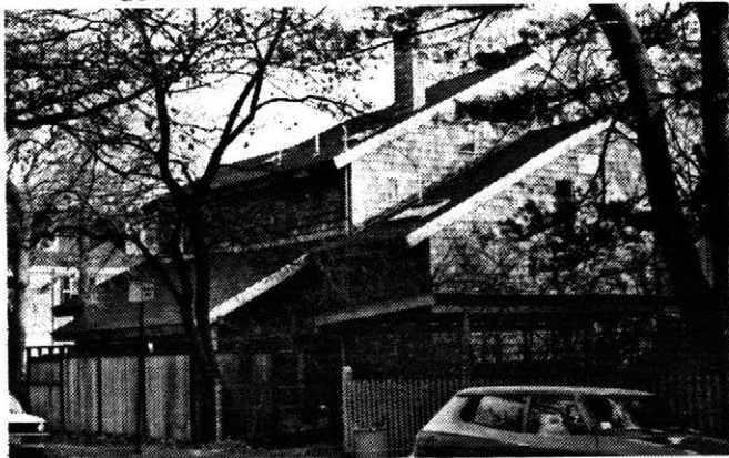
Below: North/Street side closed down and sheltered from cold
