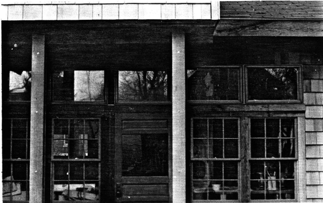
Above: Detail of south elevation
