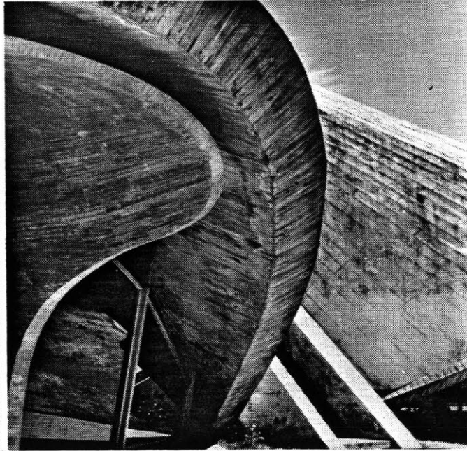
Concrete can be treated in ways that give it interesting texture. Leandro V. Loscin, architect.
