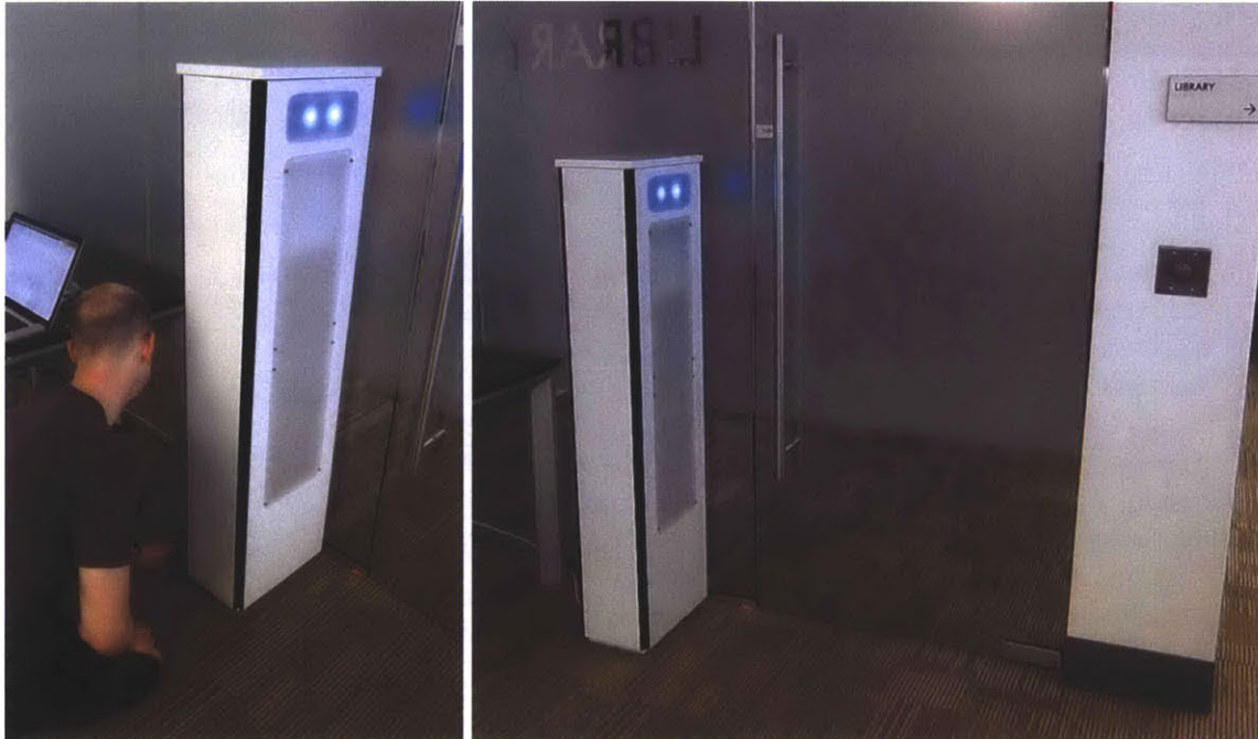
Figure 6-39. RFID Tower installation near FCAT library.
