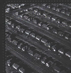
WALL AND ROOF COVERING, EN MASSE
