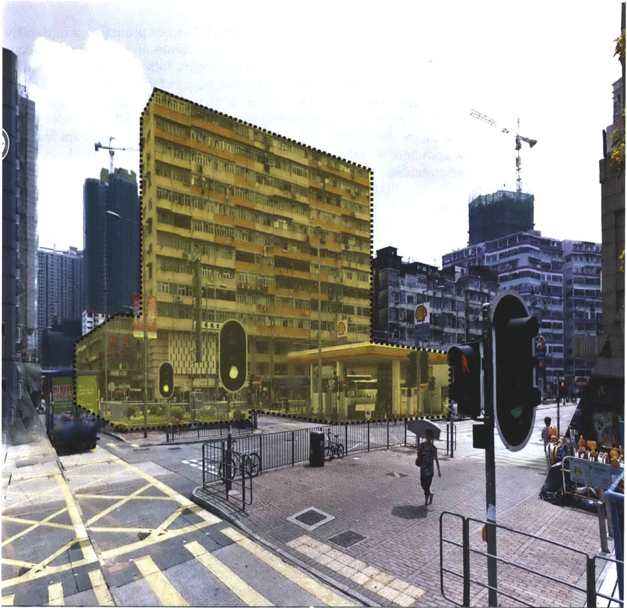
BLOCKS TO BE REDEVELOPED
