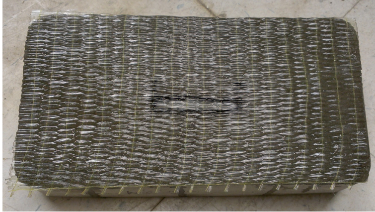
Figure 4-10: FRPP3, FRP-bonded concrete panel Size: Height 7" \times Width 13" \times Depth 4" Angled crack-like defect size: Height 0.25" \times Width 3" \times Depth 1.5", approximately 30° angle
