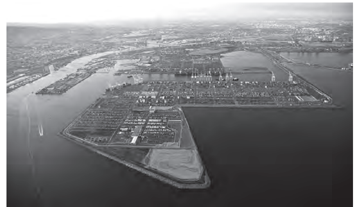
Alameda Corridor "trench" (Photo by Lane Barden) Port of LA (Photo by Noe Montes)
