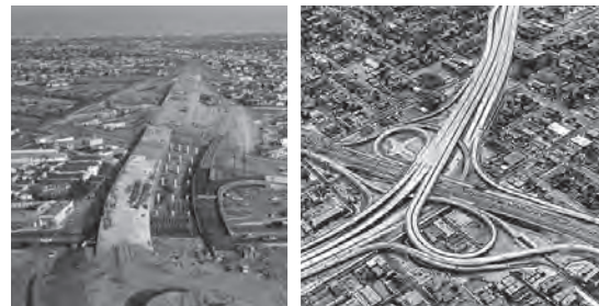
10 FWY Construction and 10-110 FWY Interchange (UCLA Historical Archive)
