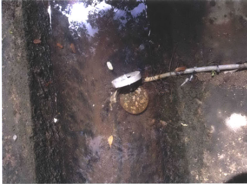
Figure 10. Coupon C2, located downstream of C1 at Lorong 8 Toa Payoh, with a vertical coupon upstream to block debris.
