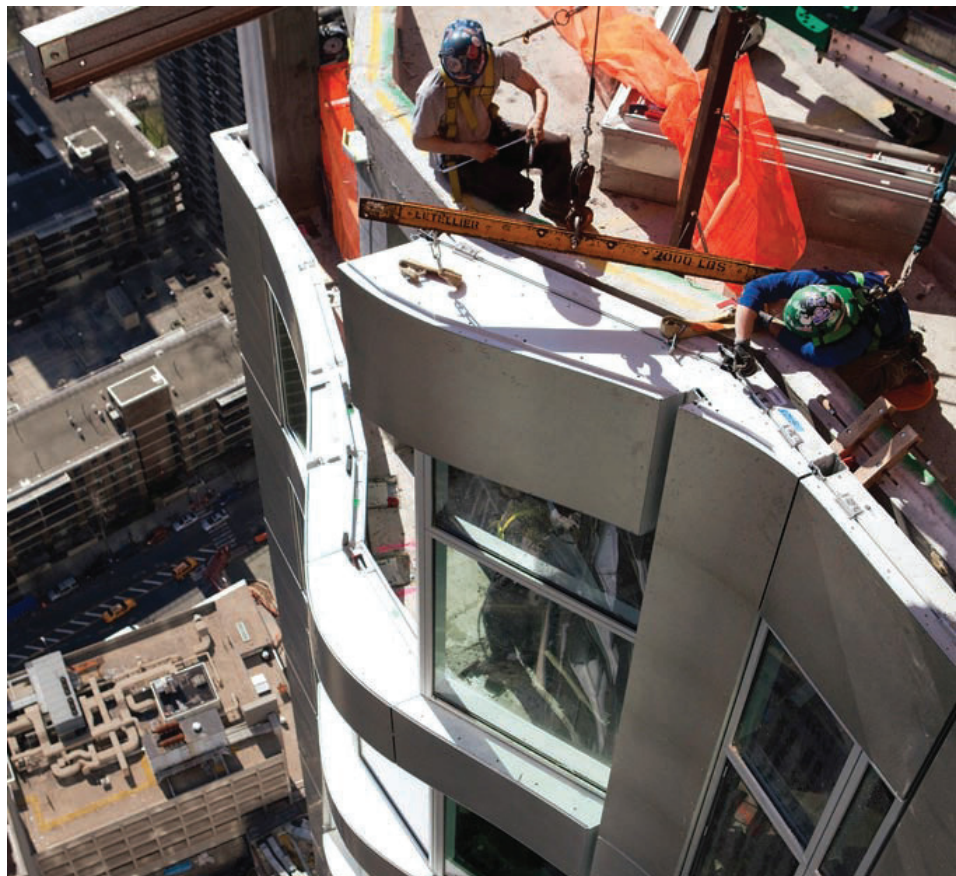
Figure 3-11: The installation of the stainless steel panels.
