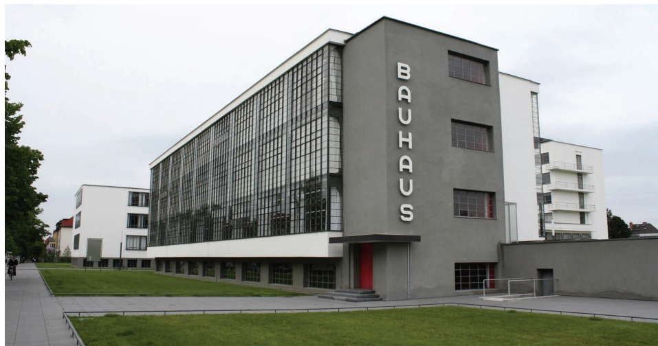
Figure 2-1: The Bauhaus in Dessau designed by Walter Gropius, 1925-1926. The curtain wall with the repetitive cast iron elements frames was prefabricated and assembled on site.
