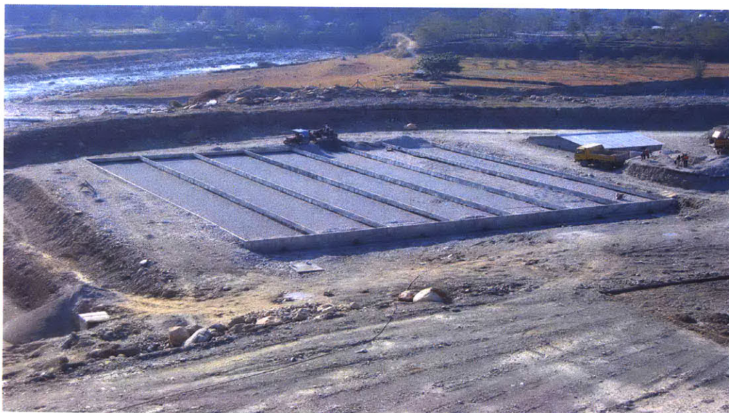
Figure 5.16: Sand Drying Bed
