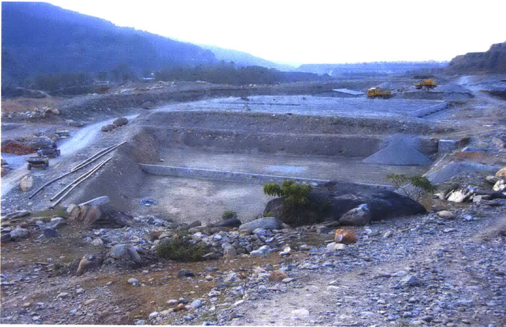
Figure 5.19: Horizontal Flow Bed
