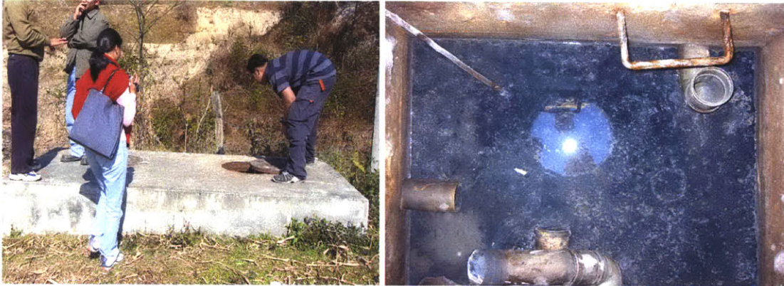
Figure 6.6: Collection Point 3 at Dhulikhel Hospital (Effluent of HFB)
