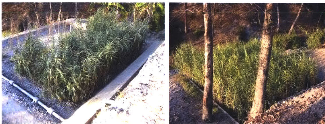
Figure 5.7: Horizontal Flow Bed (Left) and Vertical Flow Bed (Right) at SKM Hospital
