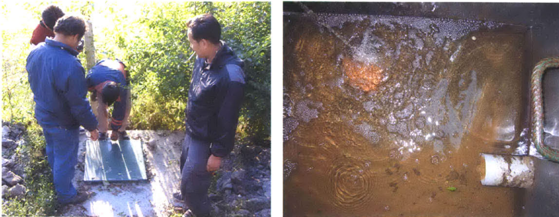
Figure 6.4: Collection Point 2 at Sushma Koirala Memorial Plastic & Reconstructive Surgery Hospital (Effluent of VFB)
