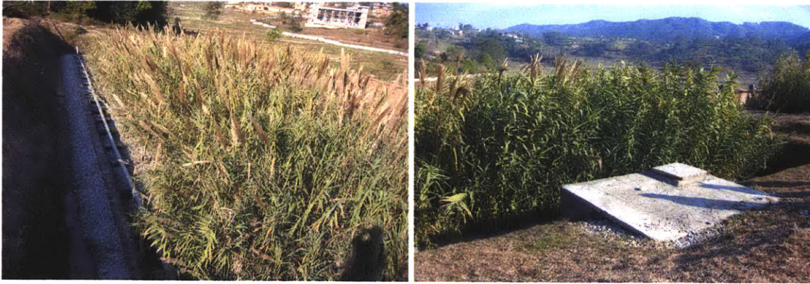
Figure 5.9: Horizontal Flow Bed (Left) and Vertical Flow Bed (Right) at SKM Hospital
