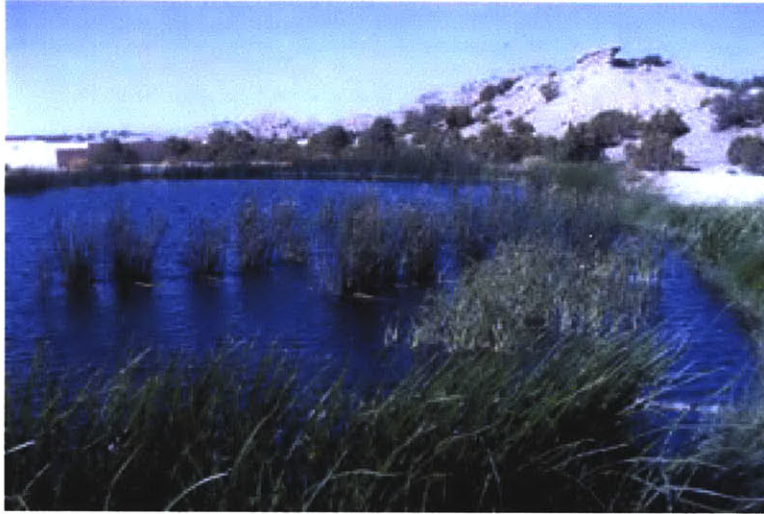
Figure 4.1: Free Water Surface (FWS) Constructed Wetlands
