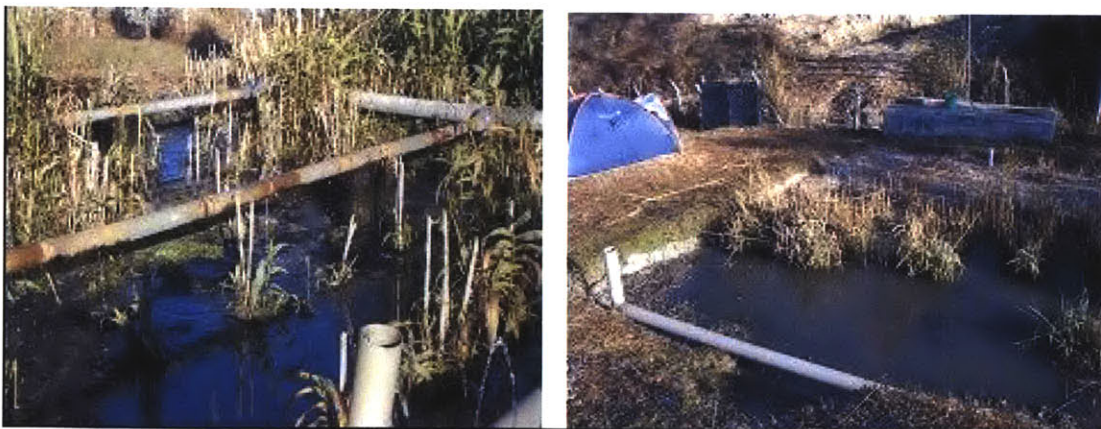
Figure 5.6: Ponding Effects on the Vertical Flow Bed (Left) and Horizontal Flow Bed (Right) at Dhulikhel Hospital Due to Sludge Accumulation.
