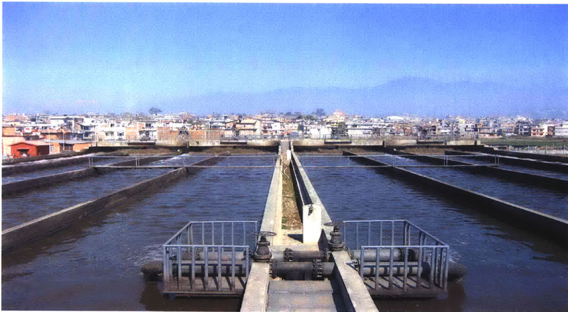
Figure 2.3: Guheshwori Wastewater Treatment Plant.
