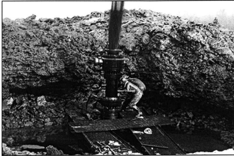
Figure 2.2: Blowout due to under balance of mudweight in borehole.<sup>3</sup>
