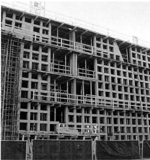
Figure 180 Exterior view of unfinished façade.
