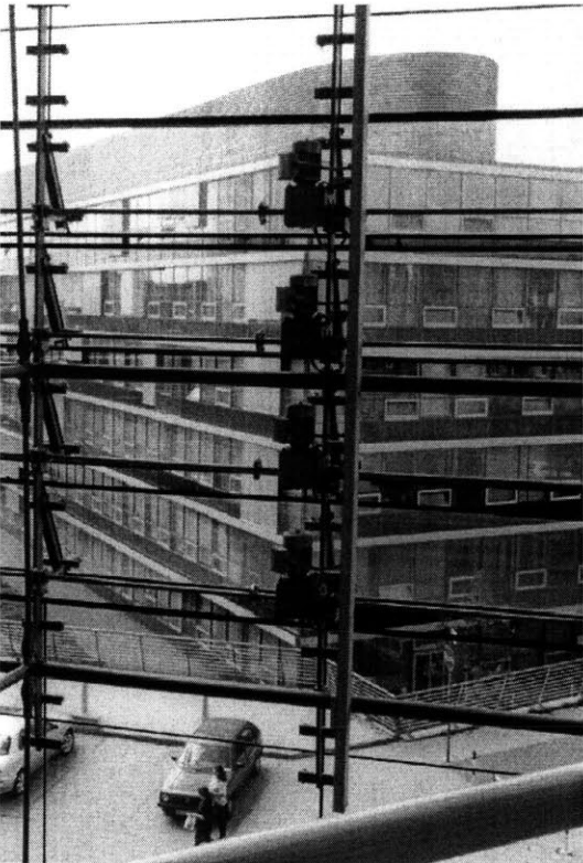
Figure 43 Lower motorized atrium windows. A similar set of windows is located at the upper portion of the atrium facades.
