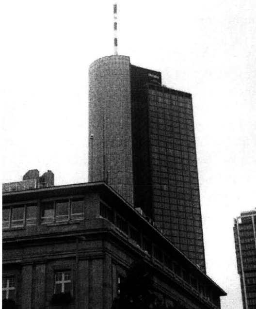
Figure 19 Exterior view. At the time this picture was taken, rain had just started falling. Note that almost all windows are closed, with the exception of some, which were in the process of closing.
