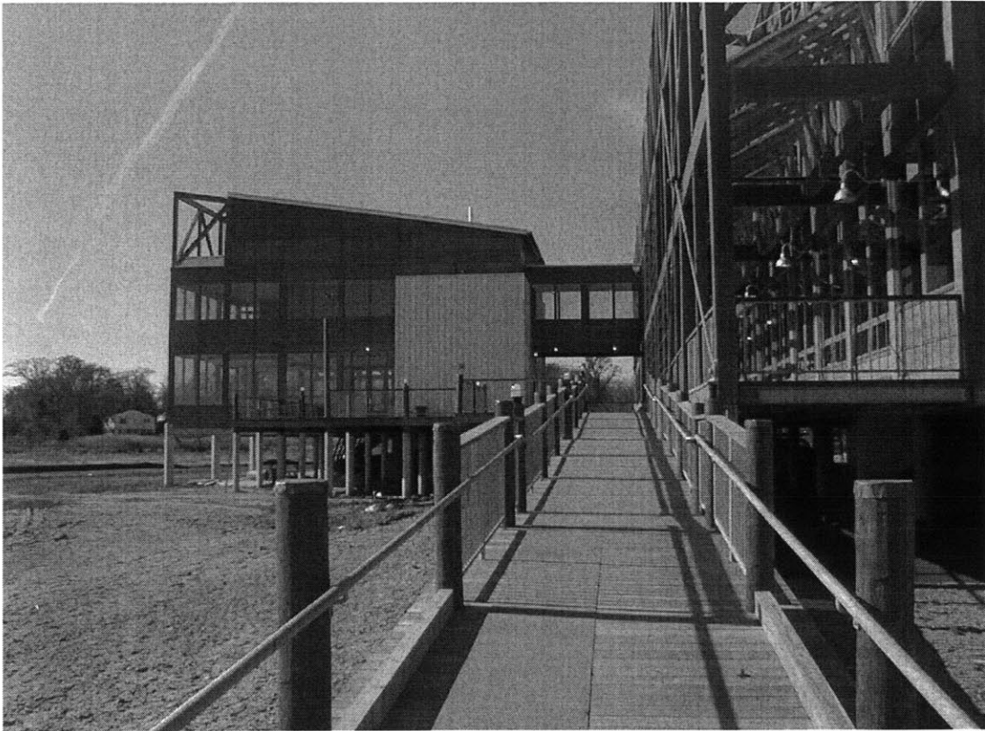
Figure 140 Conference center. The building on the left features two floors of conference rooms. There is no provision for natural ventilation in that portion of the building. On the right, the fixed wooden shading system is visible, as well as a portion of windows on the south façade.
