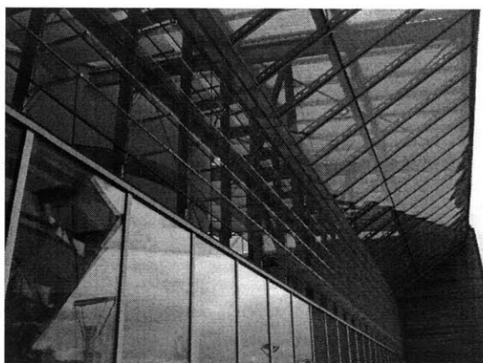
Figure 55 Operable shutters of one of the main building atriums.
