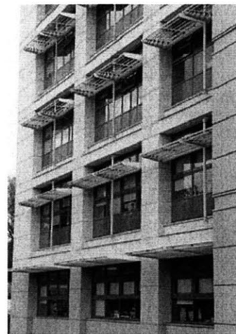
Figure 67 Outer façade. The protrusions between the top and middle operable windows act both as shades and reflective pans, directing sunlight through the uppermost window of each façade element onto the ceilings in office areas.
