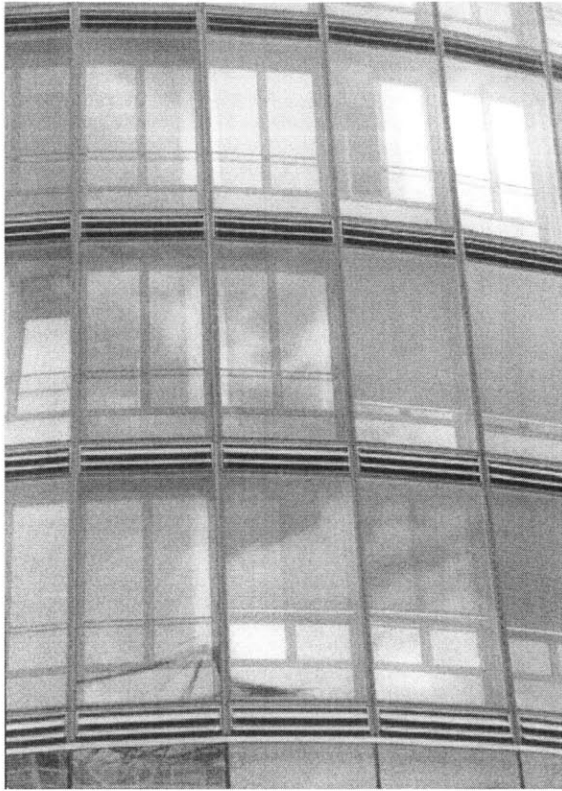
Figure 25 Partial view of façade. Note that interior windows can be tilt inwards or opened to the side. Inlet is through the channels separating each component of the façade.
