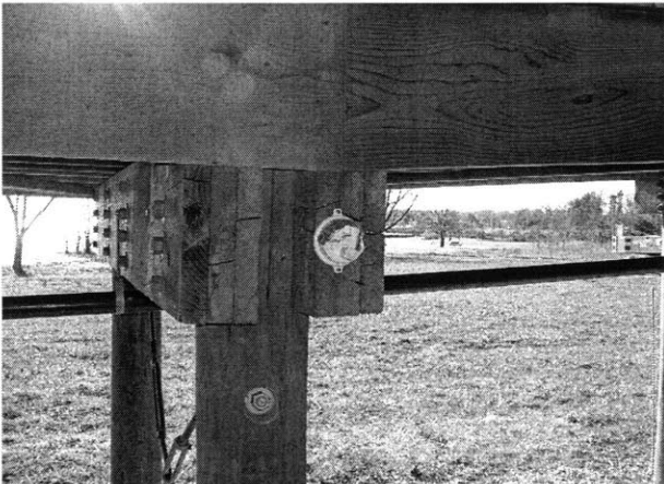
Figure 168 Outdoor temperature sensor. This sensor was mounted underneath an access ramp leading from the building to the beach. To the left of the sensor is the parking area. The sensor was shielded with reflective aluminum foil tape.
