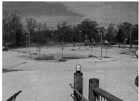
Figure 145 Parking lot. The lot is not paved to allow runoff to sink into the ground and run into specially designed collection areas.
