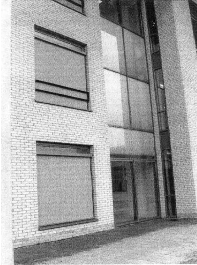
Figure 10 Exterior detail view. The shaded windows open into offices. The airflow path in the building is through the small windows above the shading, through transom windows into the hallway, and then into atriums like the one seen on the right side of the picture.
