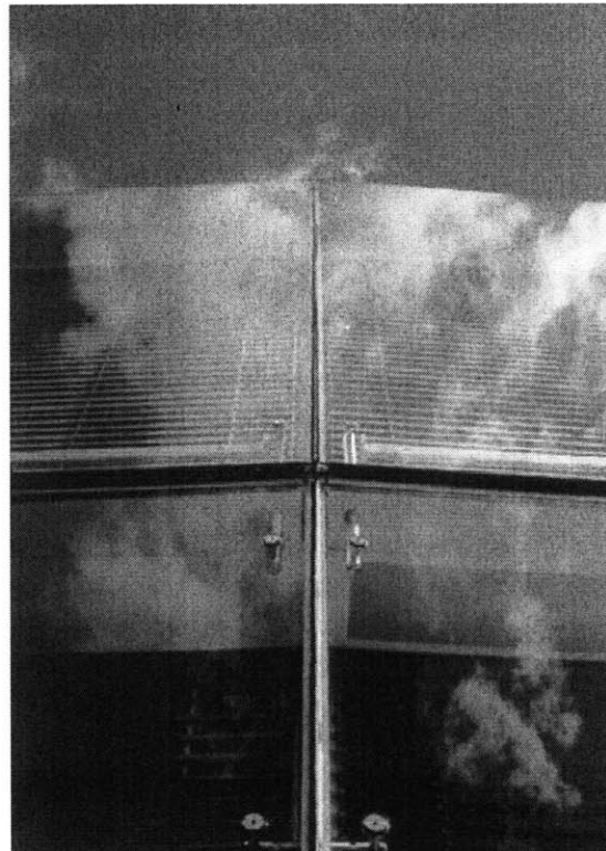
Figure 30 Actual view of façade element. From afar, the RWE tower appears to be a perfect circle, yet it is actually a 50-side polygon. The minimalist glass mounts allow for a unobstructed and complete floor to ceiling view in each room.
