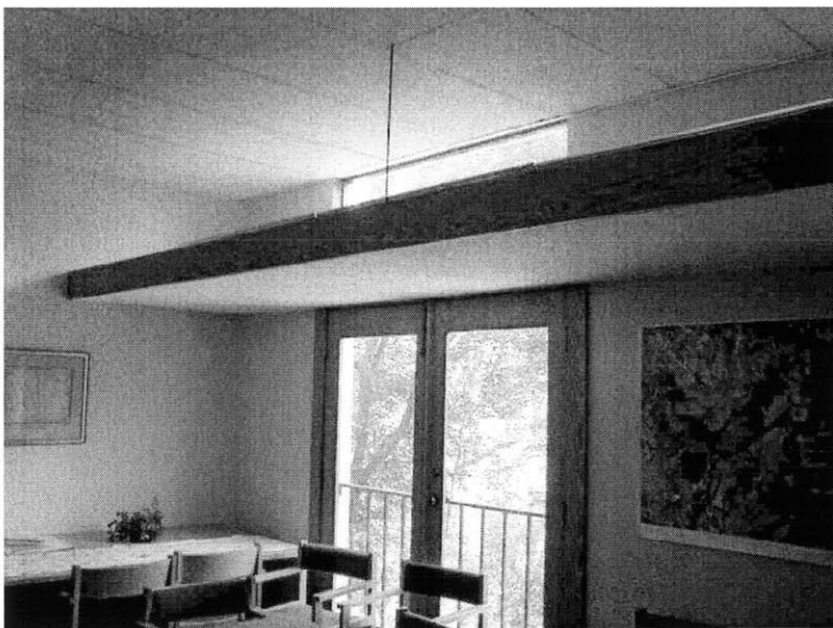
Figure 103 Conference room. Note the amount of natural daylight cast on the walls and ceiling of the space. A reflective fabric in the light pan bounces light from the upper windows onto the ceiling, to minimize artificial lighting requirements.
