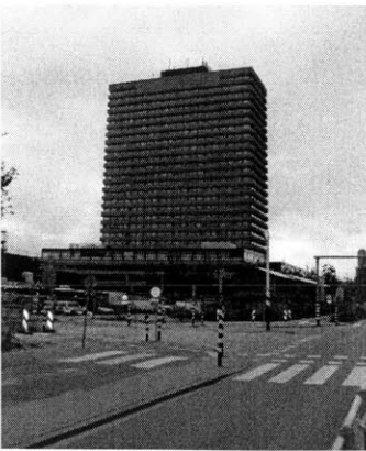
Figure 45 Exterior view of tower building.
