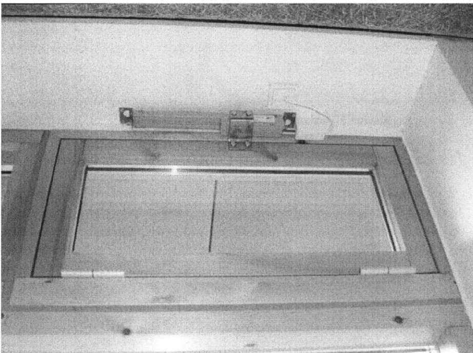
Figure 15 Top-level motorized window. The mechanism consists of a chain that winds out and in. In this case, the designer decided to expose the mechanism to give users a significant visual cue that the window is motorized.
