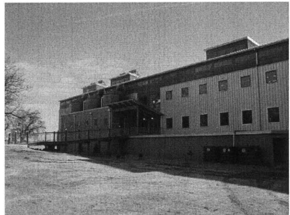
Figure 139 Another view of the north façade. Note the operable clerestory windows located on the roof. The main entrance is located at the center of the building.
