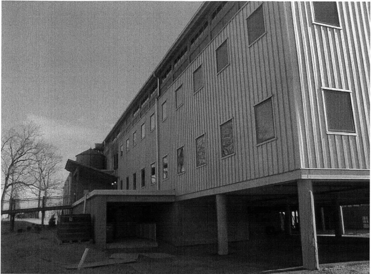
Figure 143 North façade. Some rainwater collecting cisterns are visible in this photo. All windows are operable using individual hand cranks. The space underneath the building houses approximately fifty parking spaces.
