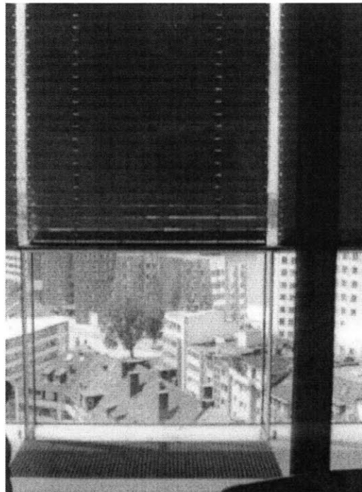
Figure 41 View of double-skin façade from the inside of a typical office.
