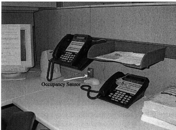
Figure 155 Workstation occupancy sensor. Each workstation features a sensor which automatically shuts off the computer monitor and task lighting when movement is not detected for fifteen minutes.
