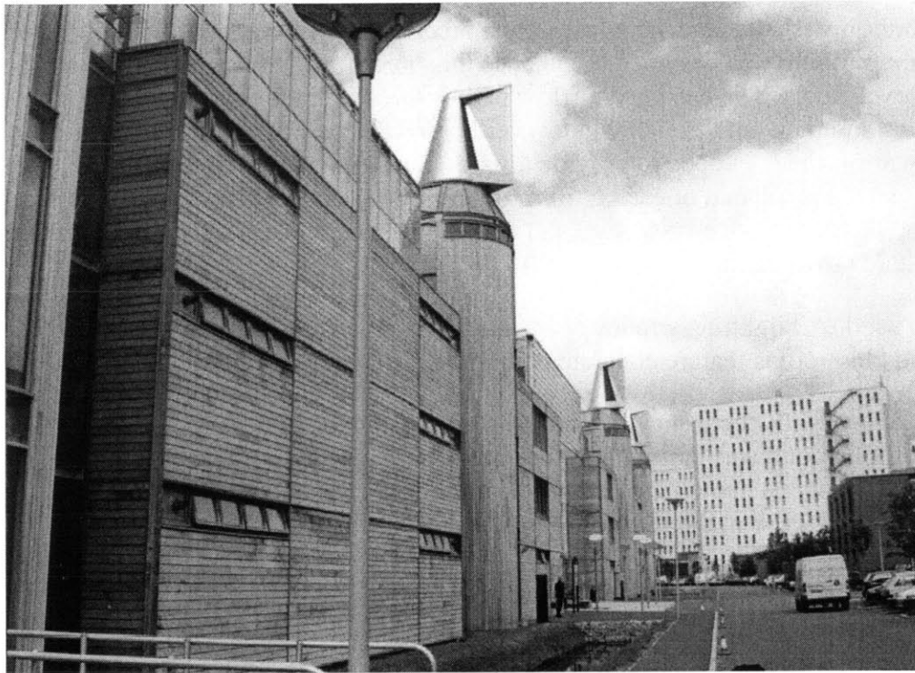
Figure 58 Backside of main campus building. The vertical wind sails can rotate to provide optimal exhaust of air from the front of the building. The small windows on the left open into restrooms and kitchen facilities.
