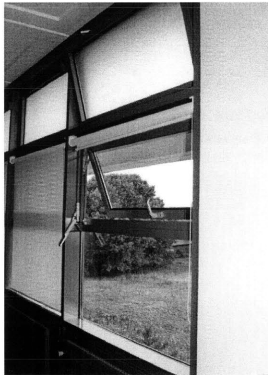
Figure 71 Office façade to outside. Note the lowered shading device on the left window. The top tilt window is frosted to smooth out sunlight and thus reduce glare. Both the top and middle windows are manually operated.
