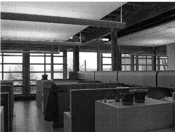
Figure 152 View of south façade from first floor east office area. Portions of the ceiling were left open for cost savings.
