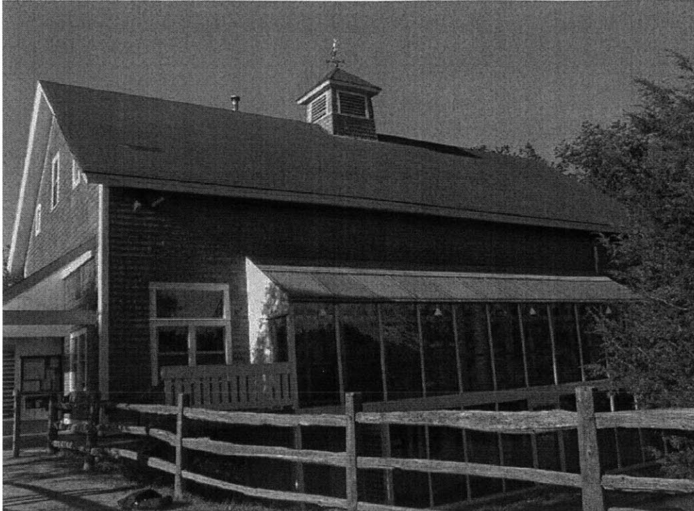
Figure 91 South façade. The glass enclosure retains heat during the winter. It is ventilated during the summer through use of two full-size doors. The cupola on the roof allows hot air to exhaust from the attic spaces.
