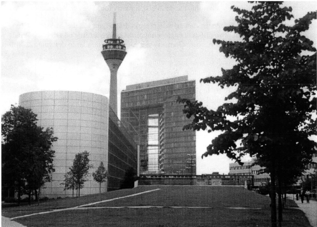
Figure 38 Exterior view. Note the atrium in the center. The top three floors are served by a smaller atrium. Windows at the bottom and top of the larger atrium façade allow for stack ventilation.
