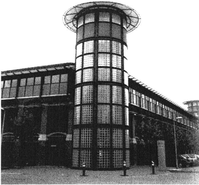
Figure 50 “Mushroom” tower. These towers are used to provide stack ventilation to the lower three floors. The roof of the tower is opened automatically when indoor temperatures have gone past a certain setpoint.
