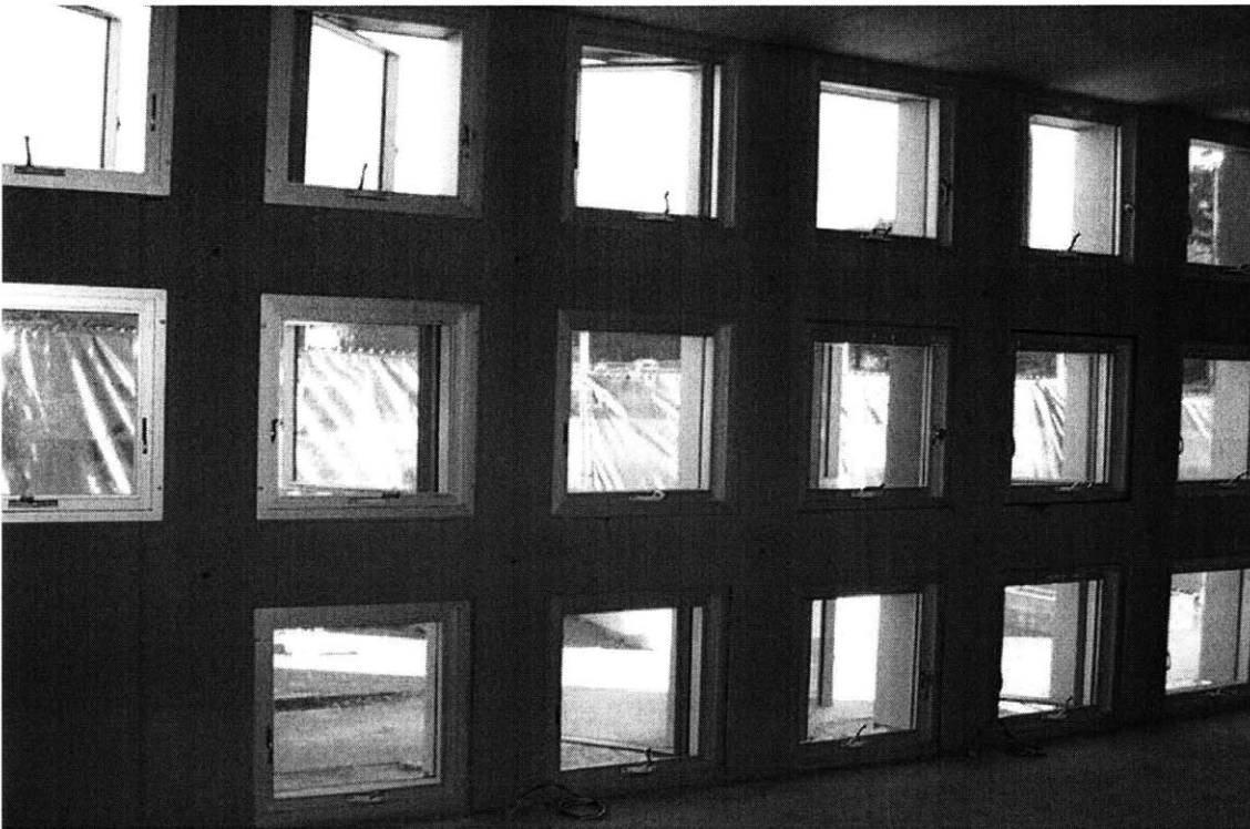
Figure 178 Interior view of windows in a double room.
