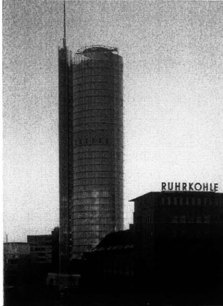
Figure 27 Exterior view at night. The rectangular shaft on the left of the circular portion of the tower houses 4 elevators for best use of space.
