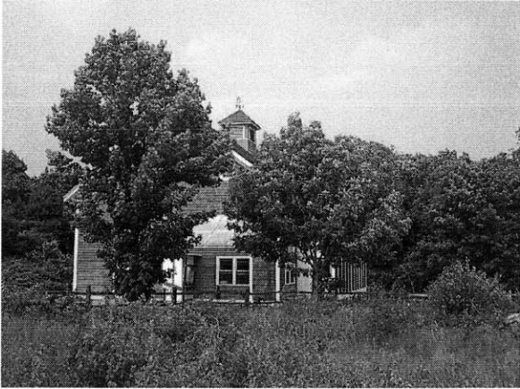
Figure 95 West façade from open field.
