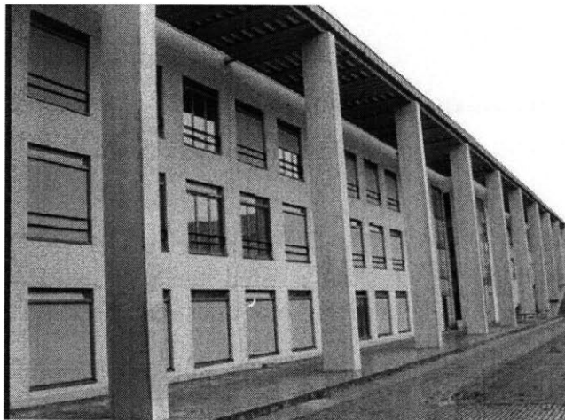
Figure 9 Exterior view. Exterior shading is automatically lowered during non-academic times for security and energy saving reasons. The windows above each shade can be operated by motor.
