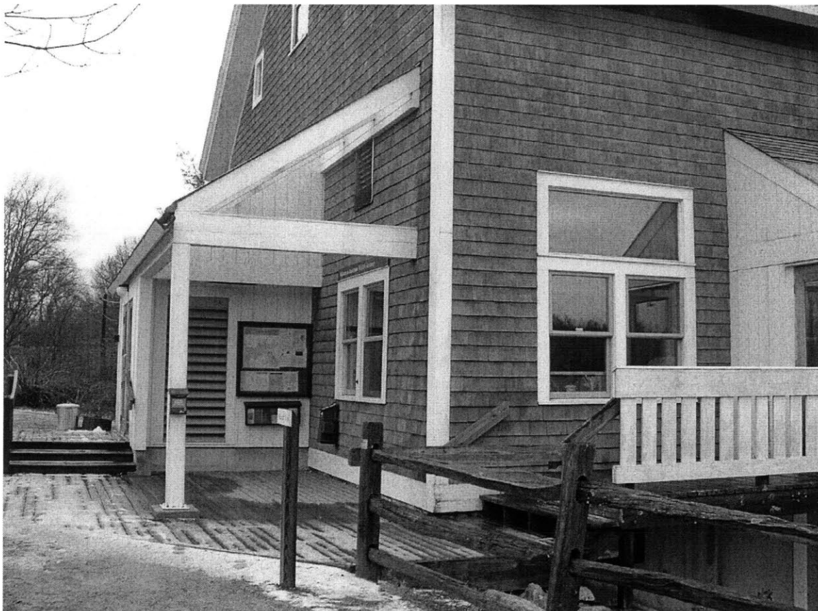
Figure 100 Southeast corner. Note the overhang on the west façade, which provides sun shading. The overhang was also designed to channel wind into the building. Also, note the louvered door for night ventilation.
