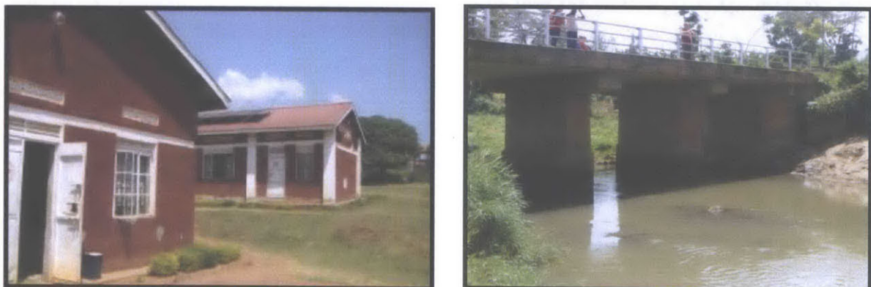
Figure 2-5: Uganda Red Cross Society Bubulo Branch (left) and the Bridge Near Bubulo Red Cross Office (right)
