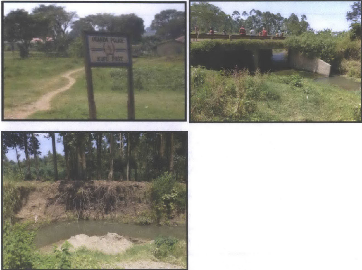
Figure 2-6: Uganda Kufu Police Post (top left), Kufu Bridge (top right), and sand mining and eroded banks adjacent to Kufu Bridge (bottom)
