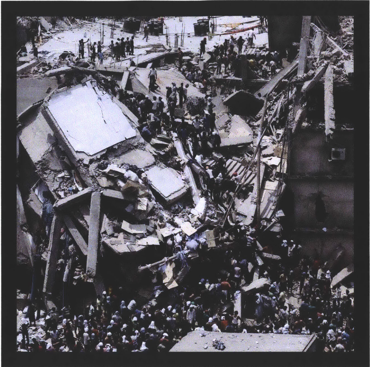
New Crimes BANGLADESH FACTORY COLLAPSE
