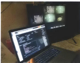
Figure 39: Control room and operator interface
