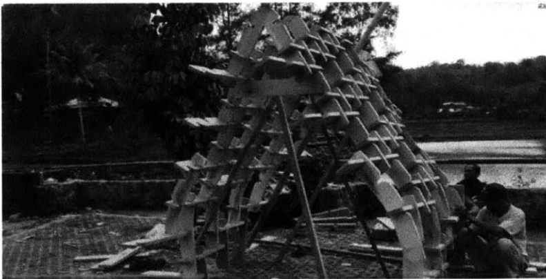
Figure 68. The Mock Up Installation
