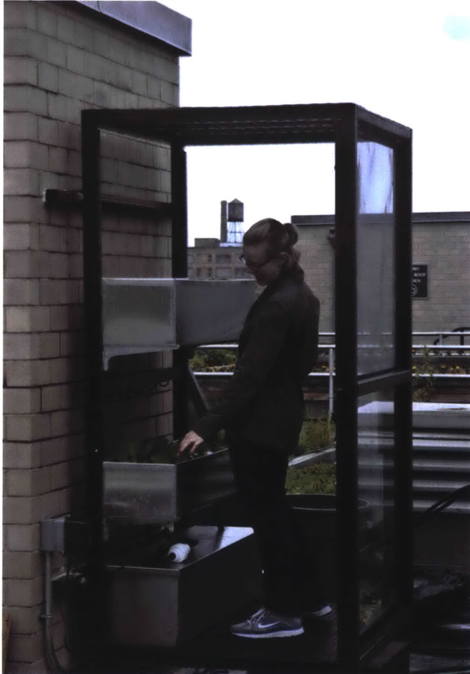
Figure 9.1 FaçadeFarm in collaboration with Fluxxlab, Boswyk Farms and the New York City Parks Department, is a prototype for a prefabricated farming module to be attached to the façade of new building construction. Image courtesy of Lee Mandel
